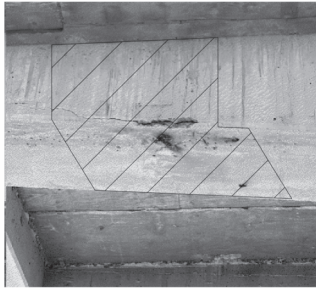
CONCRETE REPAIR PHOTO SHOWING LOCATION OF REPAIR
