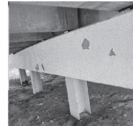
EXISTING STEEL PILES
