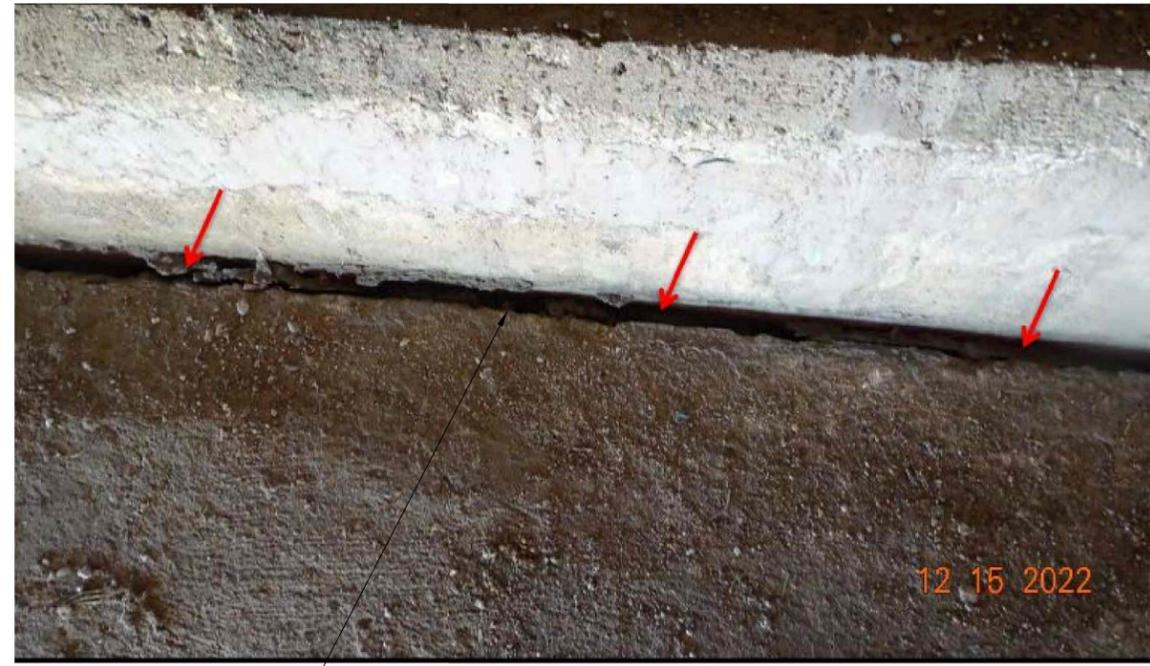
CLEANING AND SEALING EXIST JOINTS (CL 7) =79 LF
