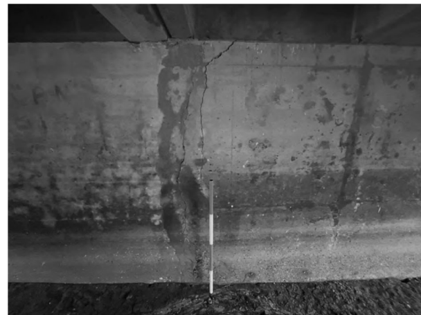
CONC STR REPAIR (VERTICAL & OVERHEAD) NORTH ABUTMENT EST @ 15 SF
