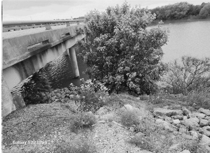
WEST SIDE LOOKING SOUTH
