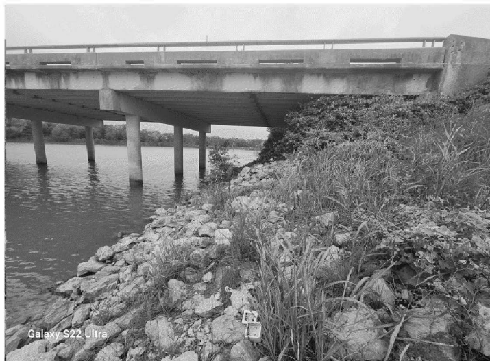
EAST SIDE LOOKING WEST
