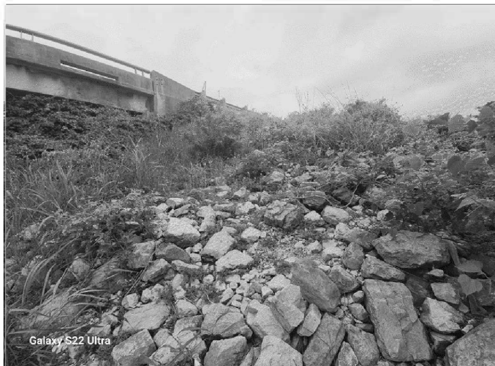
EAST SIDE LOOKING NORTH
