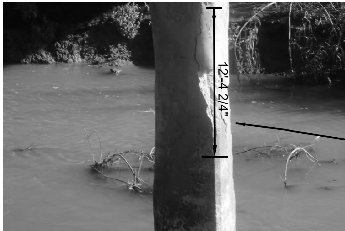
REPAIR 1 NBI: 21-109-0-1804-01-002 BENTS 2 & 3 FRACTURES IN PILES
