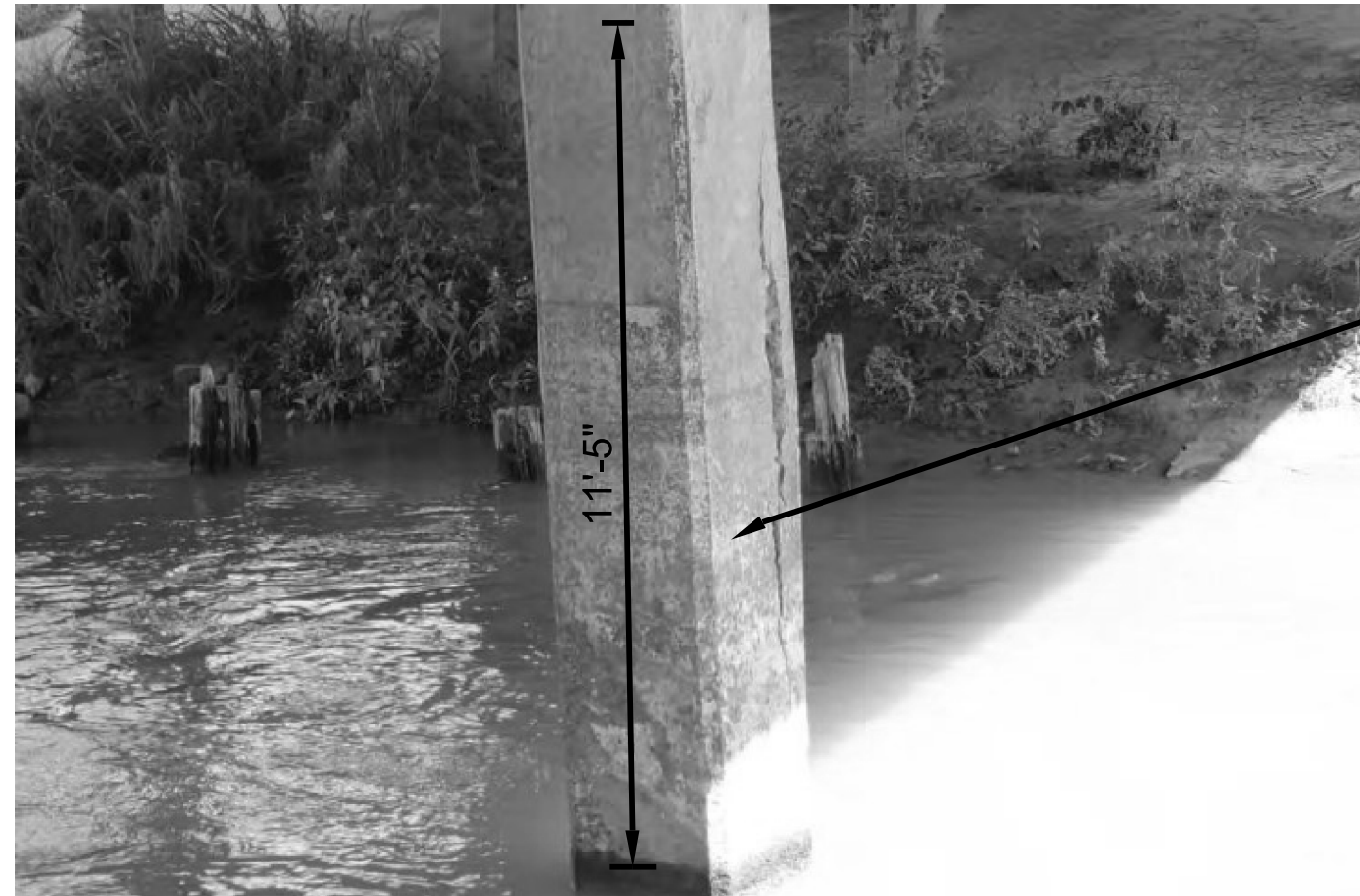
REPAIR 5 NBI: 21-109-0-1804-01-002 CRACK IN 4TH PILE FROM THE EAST IN BENT 3 LOOKING SOUTH EAST
