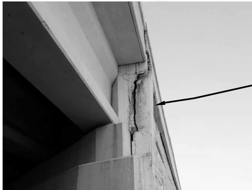
REPAIR 6 NBI: 21-031-0-0039-07-366 Coping of retaining wall at North bridge corner at NW backwall
