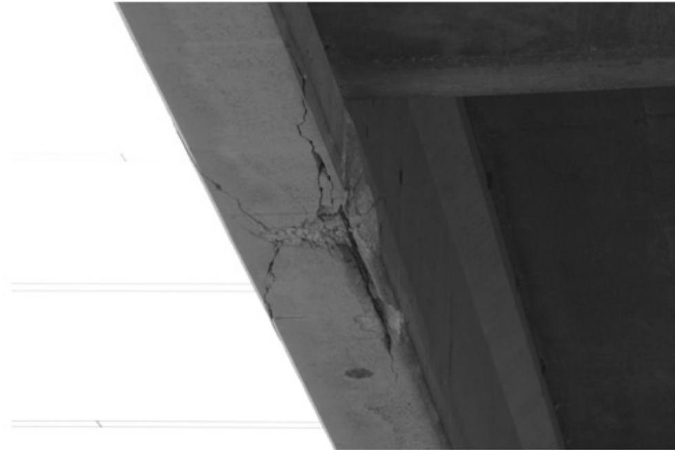
PHOTO 2. - EAST BEAM OF SPAN #2, FROM SOUTH.
