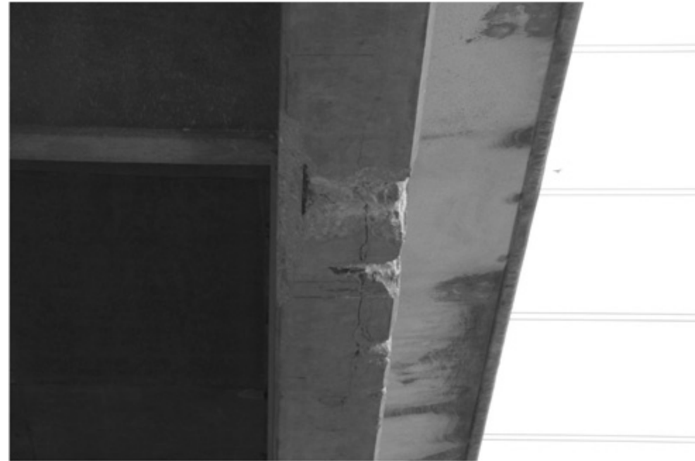
PHOTO 1. - WEST BEAM OF SPAN #2, FROM SOUTH.
