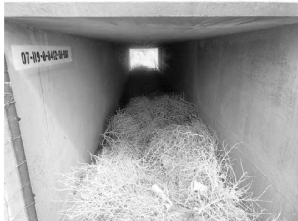
PHOTO 1. - TYPICAL DEBRIS BUILD UP IN BARRELS.
