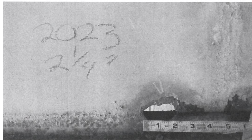
REPAIR LOCATION NO. 2 ~ BEAM END 3 FROM WEST
