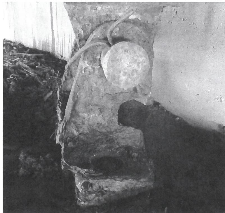
BEARING AT BEAM 3 AT NORTHWEST ABUTMENT
