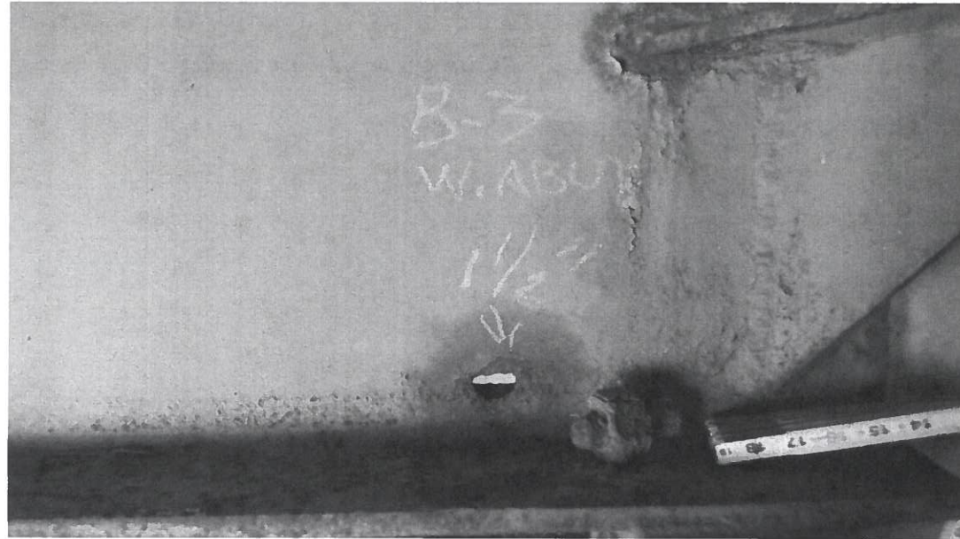
REPAIR LOCATION NO. 2 ~ BEAM END 3 FROM WEST
