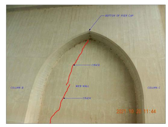
CRACK IN WEST FACE OF WEB WALL AT PIER 2 CONCRETE CRACK REPAIR (EPOXY INJECTION)
