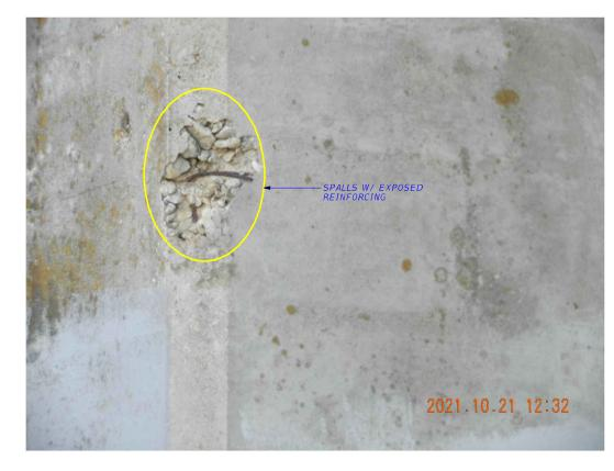
SPALL (EXPOSED REINFORCING) AT NW CORNER ABUTMENT 2
