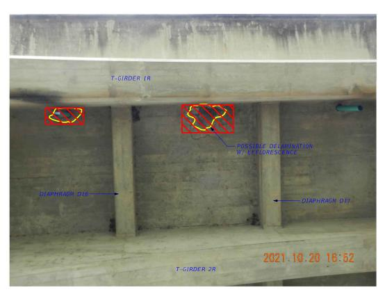
DELAMINATION (SPALL) AT UNDERSIDE OF DECK IN SPAN 9 REPAIR AS INTERMEDIATE SPALL
