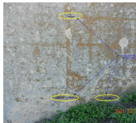
SPALLS W/EXPOSED REINFORCING (NORTH WING ABUTMENT 1)
