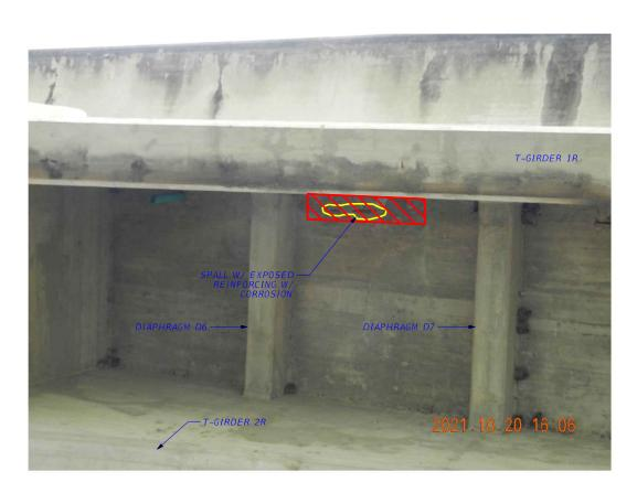
SPALL W/ EXPOSED REINFORCING UNDERSIDE OF DECK IN SPAN 8 REPAIR AS INTERMEDIATE SPALL
