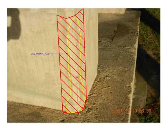
CRACK W/DELAMINATION/SPALL AT SE CORNER COLUMN C AT BENT 4 REPAIR AS INTERMEDIATE SPALL
