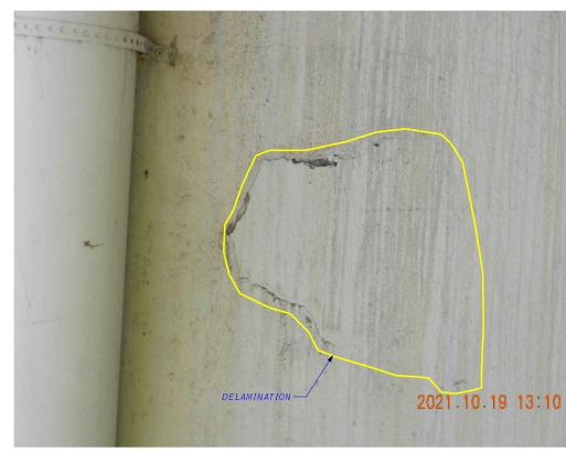
DELAMINATION (SPALL) AT ABUTMENT 1
