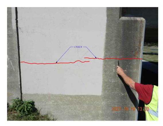
CRACKS AT SOUTH WING AT ABUTMENT 1
