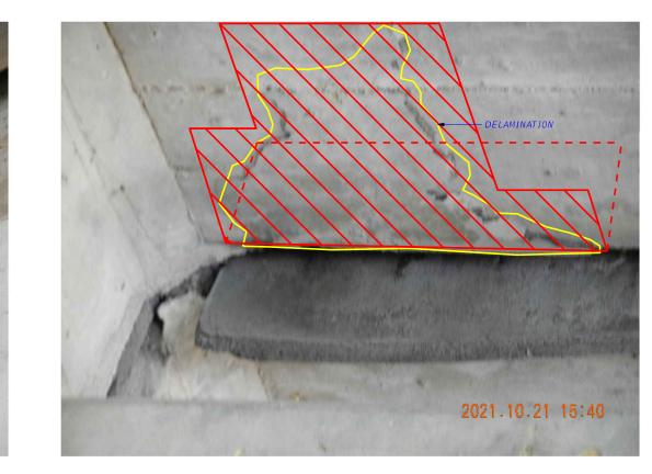
DELAMINATION (SPALL) UNDERSIDE OF DIAPHRAGM D6 IN SPAN 1 (BENT1) REPAIR AS INTERMEDIATE SPALL
