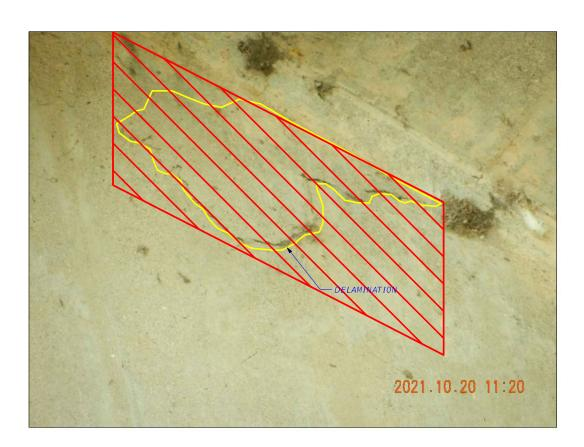
CRACK W/ DELAM/SPALL IN WEB WALL BTWN COLUMNS A & B AT PIER 1 REPAIR AS INTERMEDIATE SPALL
