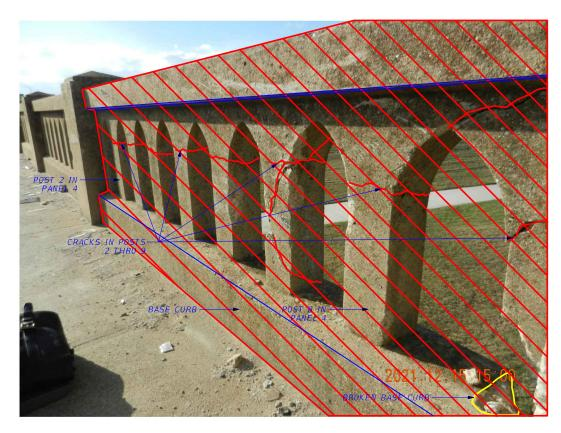
SPALL W/ EXP REINFORCING AT POST 9, PANEL 2, NORTH RAIL (SPAN 1) CRACKS POSTS 2-9 BROKEN BASE CURB IN PANEL 4, NORTH RAIL (SPAN 2)
