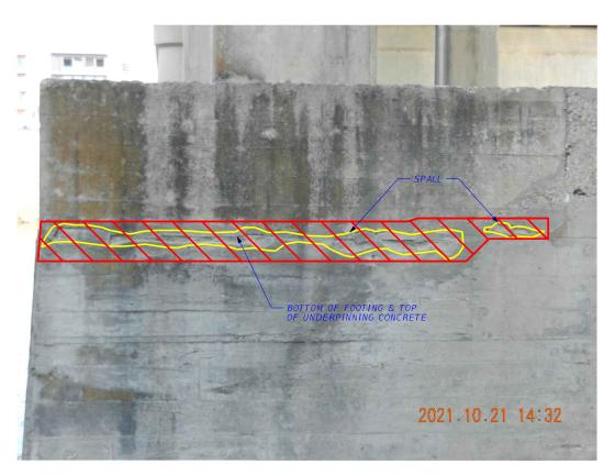
SPALLING IN WEST FACE OF FOOTING AT BENT 5 REPAIR AS MINOR OR INTERMEDIATE SPALL (DEPENDS ON DEPTH AND IF REINFORCING IS ENCOUNTERED DURING PREPARATION)
