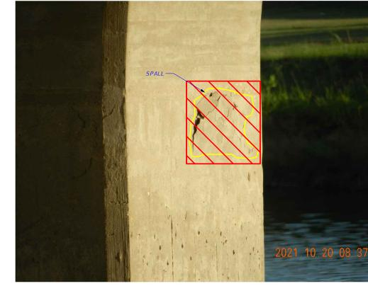
SPALL W/ POPOUT AT SOUTH FACE OF COLUMN B AT BENT 5 REPAIR AS MINOR SPALL
