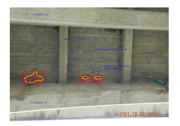
SPALLS W/ EXPOSED REINFORCING AT UNDERSIDE OF DECK IN SPAN 9 REPAIR AS INTERMEDIATE SPALL
