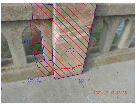
CRACK IN POST 9 AND 15" X 15" POST IN PANEL 3 IN NORTH RAIL IN SPAN 4 CONCRETE RAIL REPLACEMENT (IN-KIND) - 1.93 LF (PARTIAL PANEL 3 & 15" X 15" POST)
