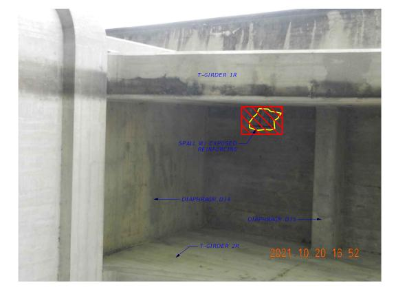
SPALL W/ EXPOSED REINFORCING AT UNDERSIDE OF DECK IN SPAN 9 REPAIR AS INTERMEDIATE SPALL
