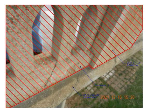
RAIL PANEL FAILURE (& DECK FAILURE) IN PANEL 1 IN NORTH RAIL IN SPAN 5 CONCRETE RAIL REPLACEMENT (IN-KIND) - 11.94 LF (PEDESTAL & PANEL 1)
