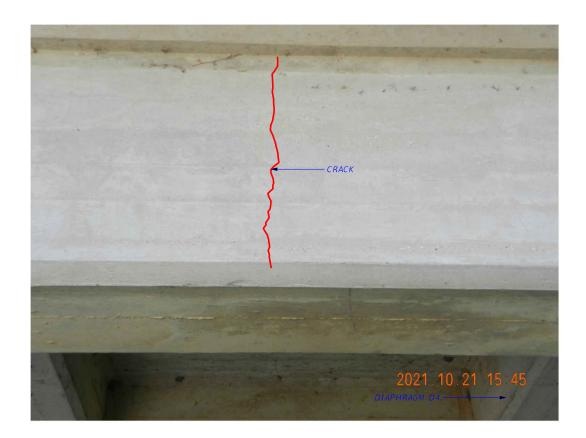
CRACK IN NORTH FACE OF T-BEAM 1L IN SPAN 1 CONCRETE CRACK REPAIR (EPOXY INJECTION)
