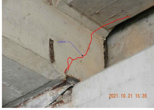
CRACK AT NORTH SIDE OF T-BEAM 2L IN SPAN 1 (ABUT 1) CONCRETE CRACK REPAIR (EPOXY INJECTION)
