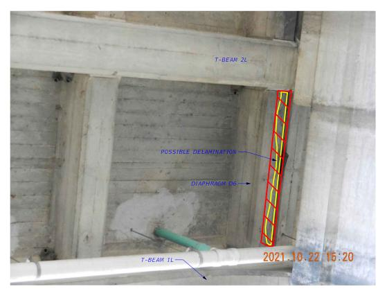
CRACKS W/ DELAM/SPALL UNDERSIDE OF DIAPHRAGM D6 IN SPAN 5
