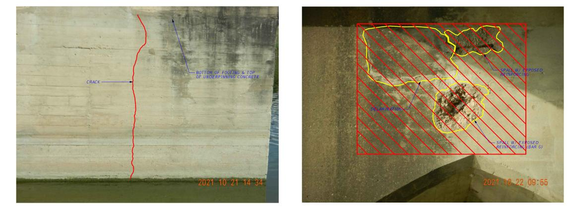
VERTICAL CRACK IN WEST FACE OF UNDERPINNING CONCRETE AT BENT 5 MAJOR SPALL W/ SEVERE CORROSION AT EAST FACE OF CAP AT BENT 7 CONCRETE CRACK REPAIR (EPOXY INJECTION) REPAIR AS MAJOR SPALL (REFER TO SHEET "BENT REPAIR BENTS 6 & 7" FOR REPAIR DETAIL")
