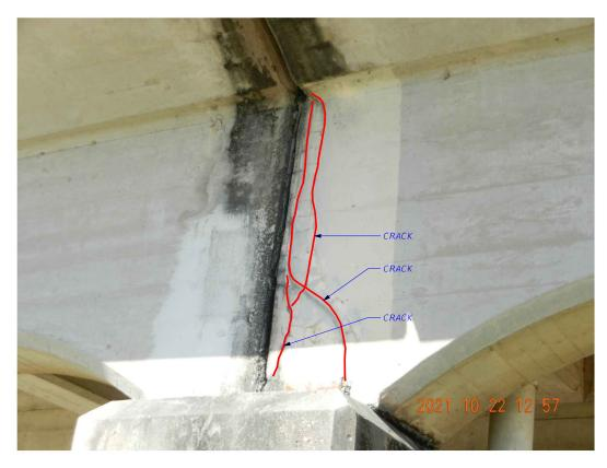
CRACKS AT SOUTH SIDE OF T-BEAM 1R IN SPAN 2 (BENT 1) CONCRETE CRACK REPAIR (EPOXY INJECTION)
