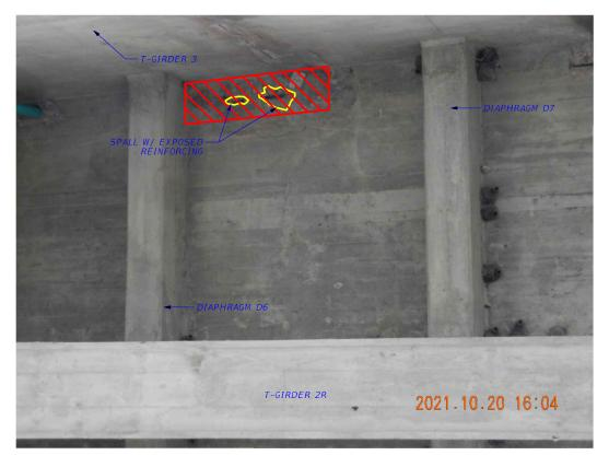
SPALL W/ EXP REINFORCING UNDERSIDE OF DECK IN SPAN 8 REPAIR AS INTERMEDIATE SPALL
