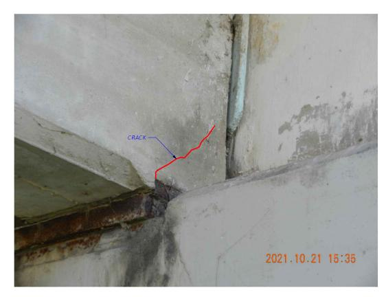
DIAGONAL CRACK IN NORTH SIDE OF T-BEAM 1L IN SPAN 1 (AT ABUT 1) CONCRETE CRACK REPAIR (EPOXY INJECTION)
