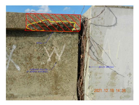
SPALL AT TOP OF NORTH WINGWALL PARAPET AT ABUTMENT 1 CONCRETE RAIL REPAIR (IN-KIND) - 2 LF (WINGWALL PANEL) REPAIR AS INTERMEDIATE SPALL
