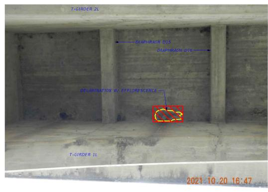
DELAMINATION (SPALL) AT UNDERSIDE OF DECK IN SPAN 9 REPAIR AS INTERMEDIATE SPALL
