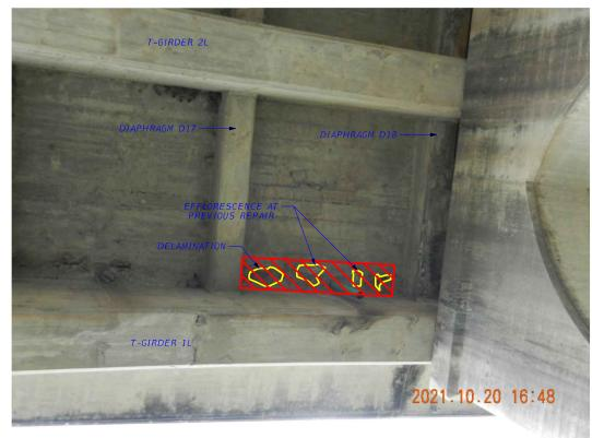
PREVIOUS REPAIR DELAMINATING AT UNDERSIDE OF DECK IN SPAN 9 REPAIR AS INTERMEDIATE SPALL
