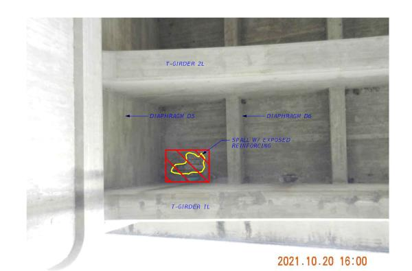
SPALL UNDERSIDE OF DECK W/ EXPOSED REINFORCING IN SPAN 8
