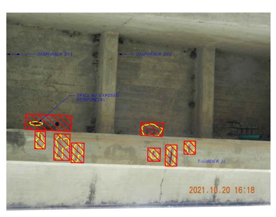
SPALL UNDERSIDE OF DECK W/ EXPOSED REINFORCING IN SPAN 8 REPAIR AS INTERMEDIATE SPALL
