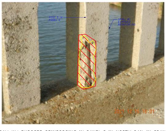
SPALL W/ EXPOSED REINFORCING IN PANEL 5 IN NORTH RAIL IN SPAN 8 CONCRETE RAIL REPAIR (IN-KIND) - 1 LF (PANEL 5) REPAIR AS MINOR SPALL (CLEAN REINFORCING, APPLY CORROSION PROTECTION COATING, EPOXY MORTAR) <u>GENERAL NOTES:</u>
