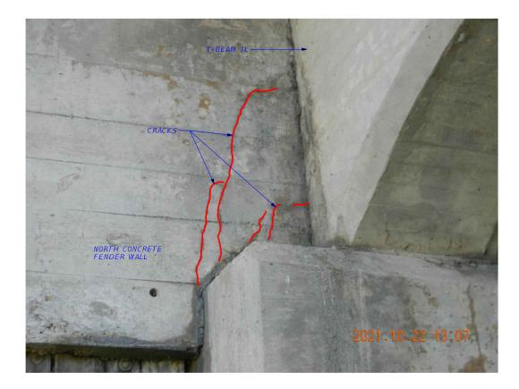
CRACKS IN W FACE OF FENDER WALL NORTH SIDE IN SPAN 2 (BENT 2) CONCRETE CRACK REPAIR (EPOXY INJECTION)
