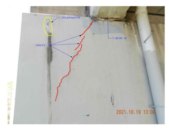
DELAMINATION AND CRACKS AT ABUTMENT 1
