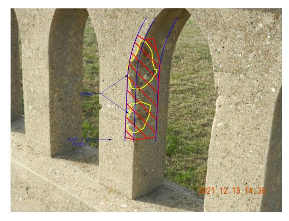
SPALLS IN 5" X 5" POSTS IN PANEL 1 IN NORTH RAIL IN SPAN 1 CONCRETE RAIL REPAIR (IN-KIND) - 1 LF (PANEL 1) REPAIR AS MINOR SPALL
