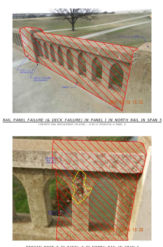
BROKEN POST 8 IN PANEL 2 IN NORTH RAIL IN SPAN 6 CONCRETE RAIL REPLACEMENT (IN-KIND) - 1.76 LF (PARTIAL PANEL 2)
