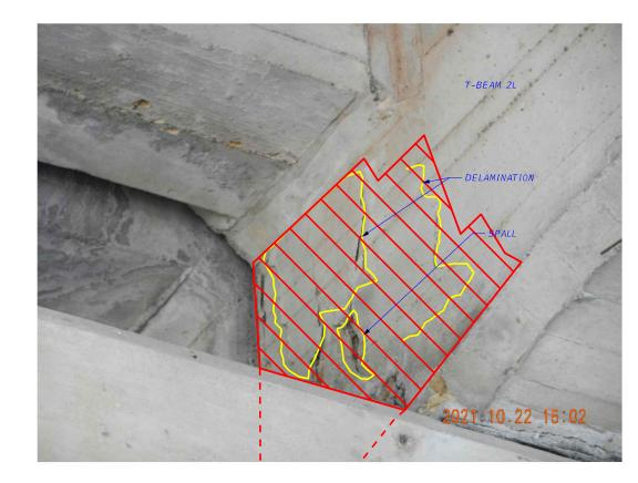
DELAMINATION/SPALLS S SIDE OF T-BEAM 2L IN SPAN 4 REPAIR AS INTERMEDIATE SPALL
