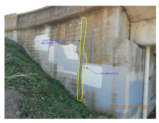
DELAMINATION (SPALL), CRACKING AT NORTH WING ABUTMENT NO 2
