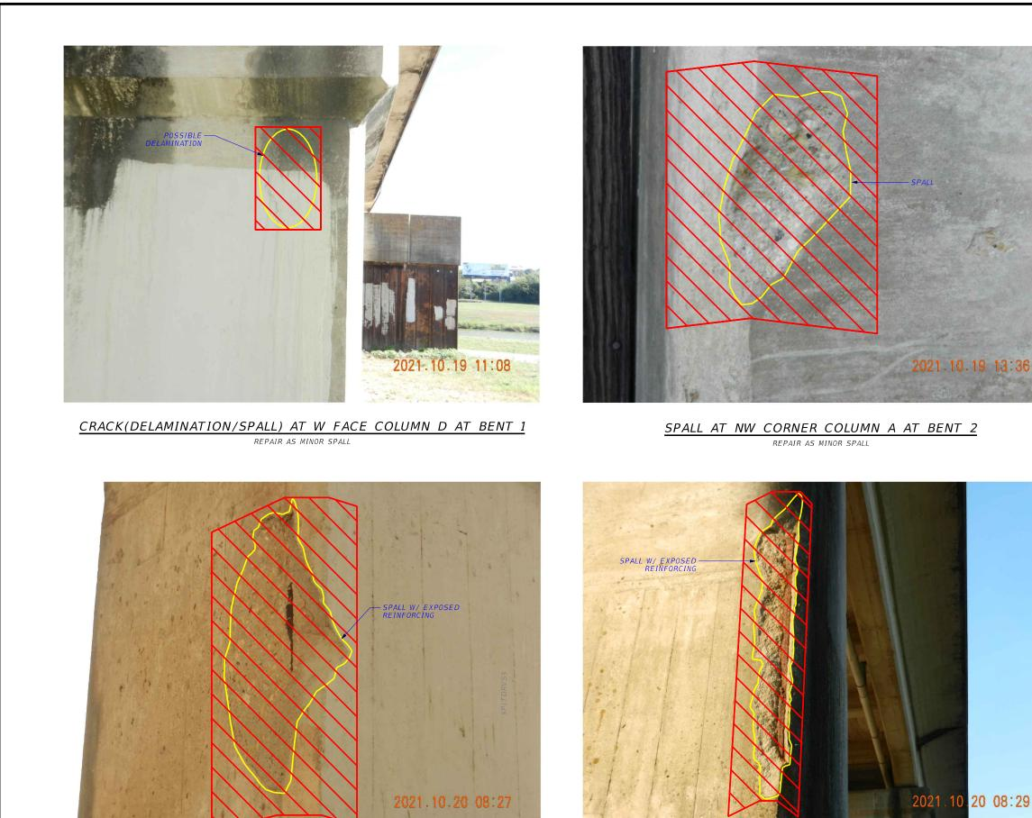
SPALL W/ EXPOSED REINFORCING AT NW CORNER COLUMN D AT BENT 4 SPALL W/ EXPOSED REINFORCING AT NE CORNER COLUMN A AT BENT 4 REPAIR AS INTERMEDIATE SPALL
