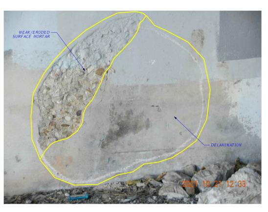
DELAMINATION (SPALL) WEST FACE ABUTMENT 2
