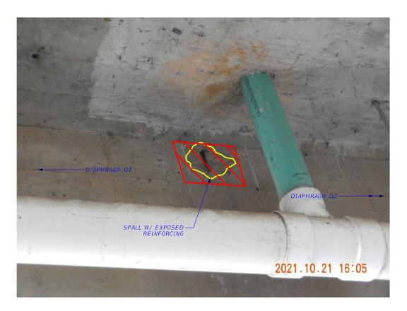
SPALL W/ EXPOSED REINFORCING IN FACE T-BEAM IR IN SPAN 1 REPAIR AS INTERMEDIATE SPALL
