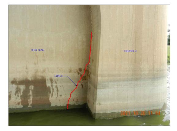
CRACK IN W FACE OF WEB WALL & N FACE COLUMN C AT PIER 2 CONCRETE CRACK REPAIR (EPOXY INJECTION)
