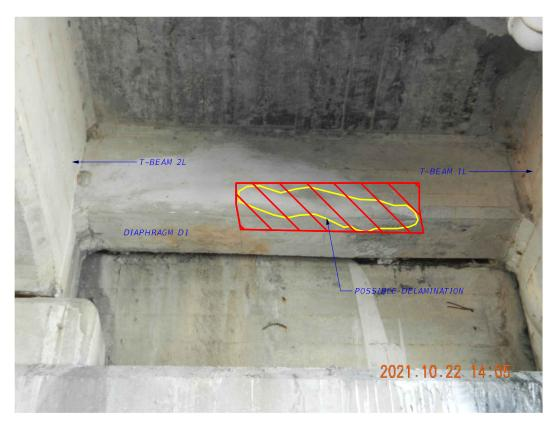
CRACK W/ DELAMINATION (SPALL) IN DIAPHRAGM D1 IN SPAN 3
