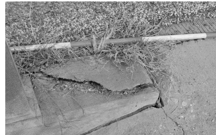
SPALL ON NORTHWEST WING WALL. PERFORM PATCHING.
