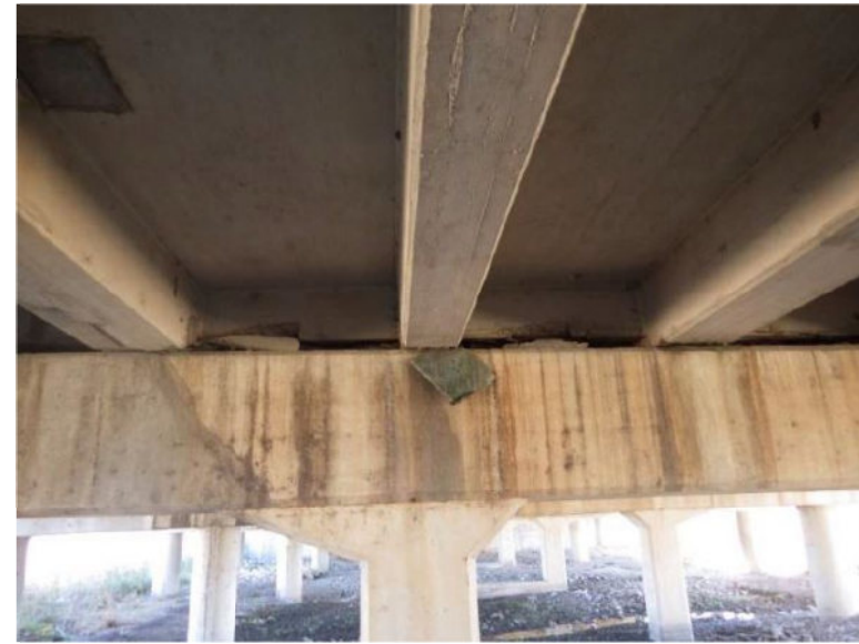
BENT 5 LOOKING NORTH
