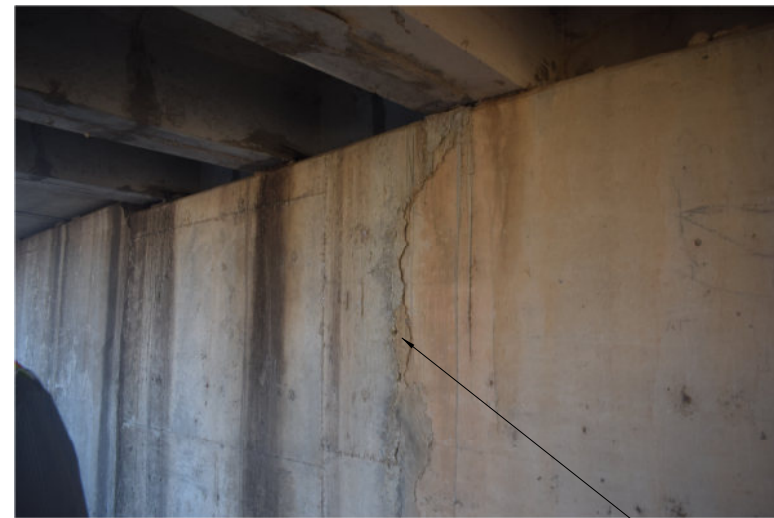
BENT 8 LOOKING NORTH
