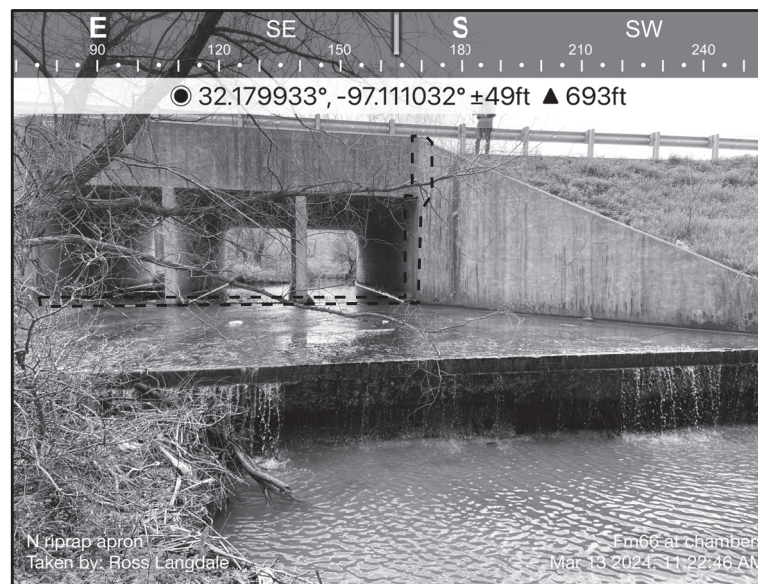
NORTH SIDE LOOKING SOUTH SHOWING LIMITS OF CONC STR / JOINT REPAIR
