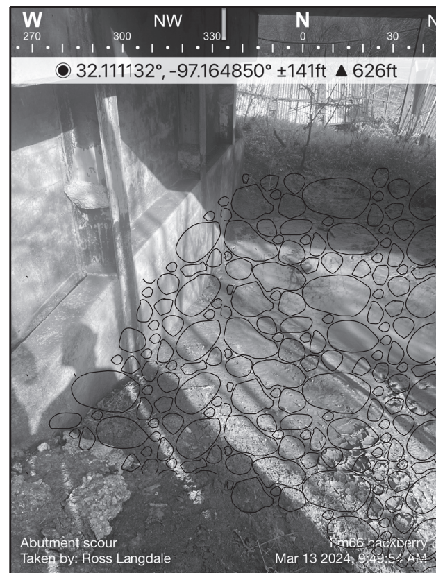
DETAIL "F" PLAN AT ABUTMENT #1 SHOWING LIMITS OF SCOUR REPAIR
