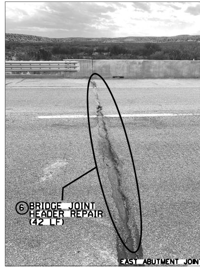
EAST ABUTMENT JOINT
