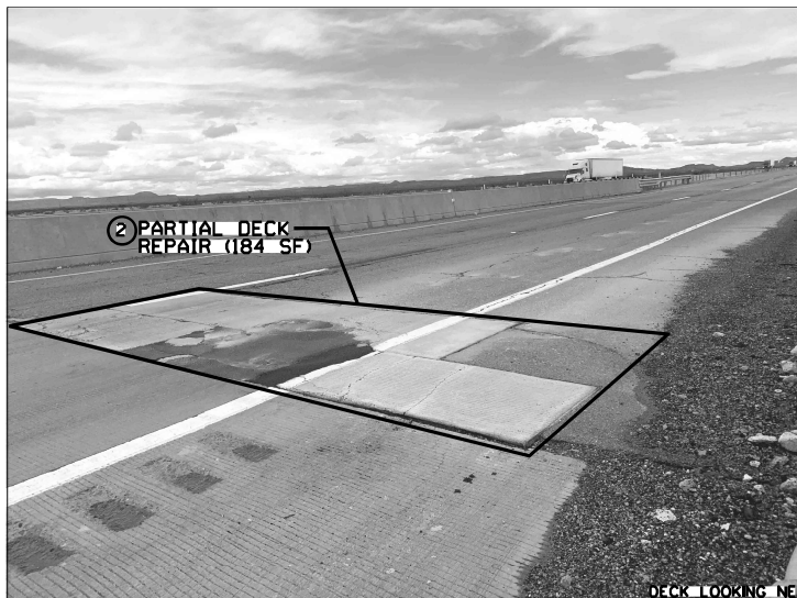
DECK LOOKING NE
