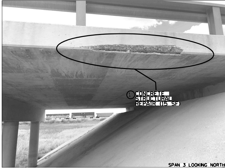
SPAN 3 LOOKING NORTH
