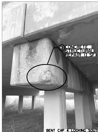
BENT CAP 4 LOOKING SOUTH
