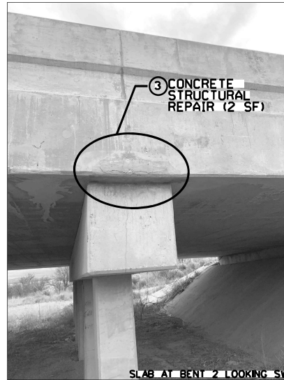
SLAB AT BENT 2 LOOKING SW
