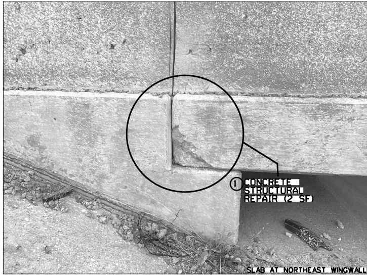
SLAB AT NORTHEAST WINGWALL
