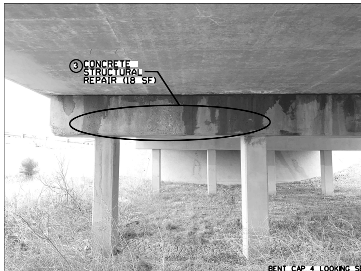
BENT CAP 4 LOOKING SE
