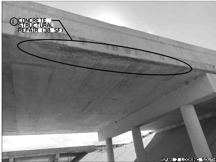
SPAN 2 LOOKING SOUTH
