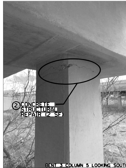
BENT 3 COLUMN 5 LOOKING SOUTH
