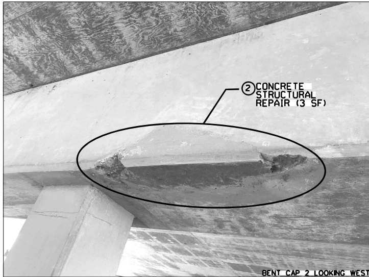
BENT CAP 2 LOOKING WEST
