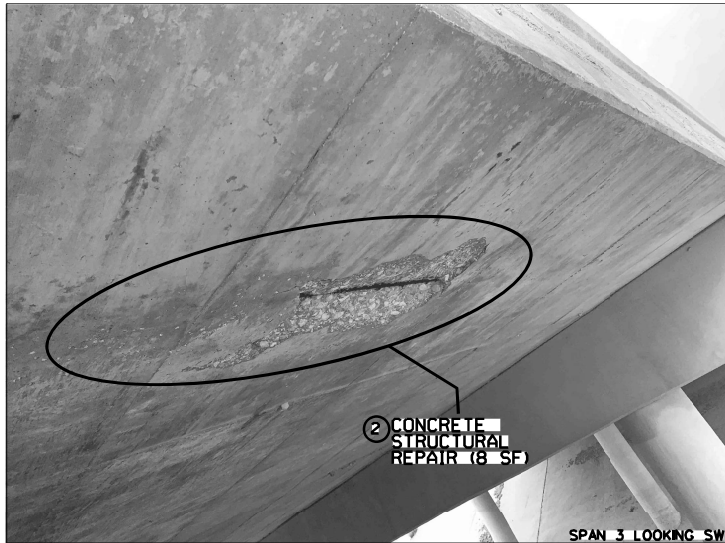
SPAN 3 LOOKING SW
