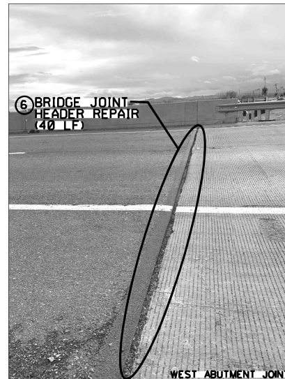
WEST ABUTMENT JOINT
