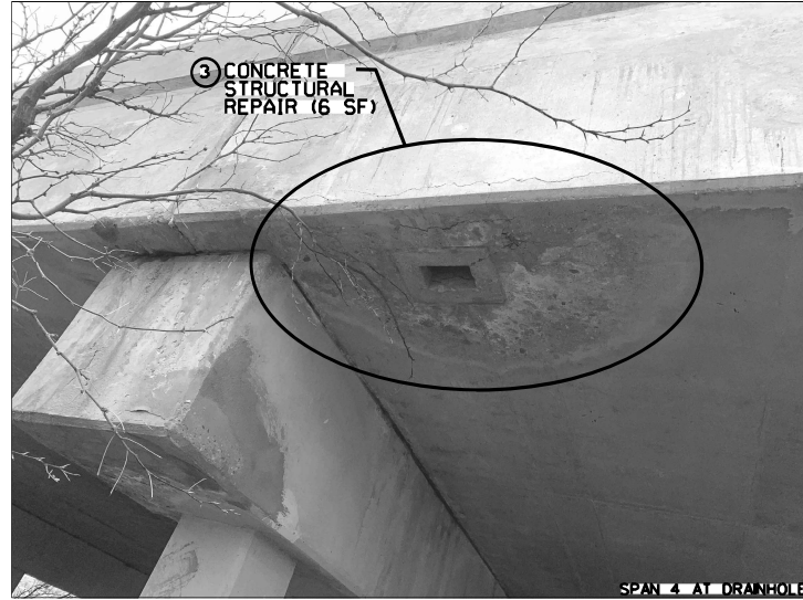
SPAN 4 AT DRAINHOLE
