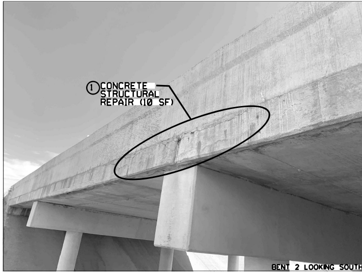
BENT 2 LOOKING SOUTH
