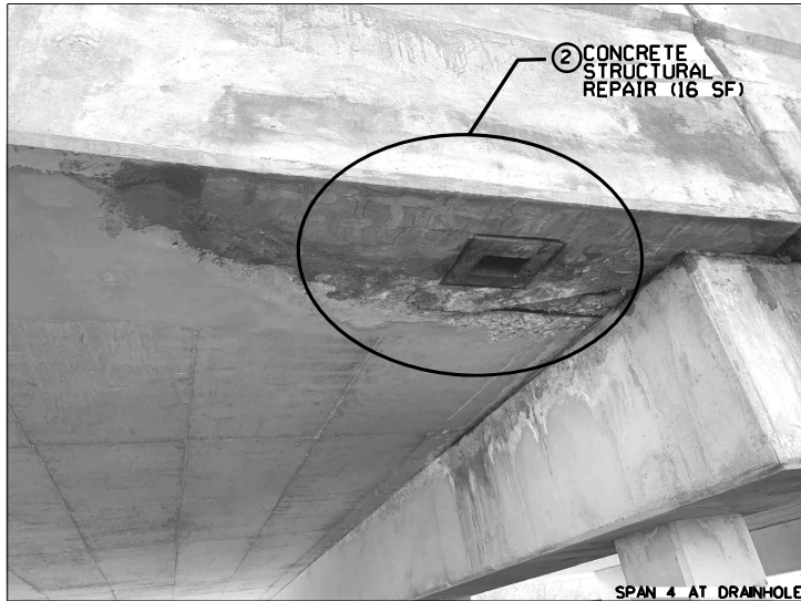
SPAN 4 AT DRAINHOLE
