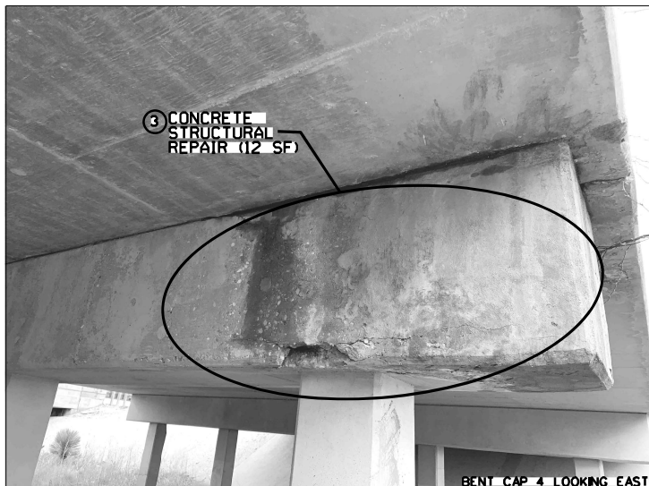
BENT CAP 4 LOOKING EAST
