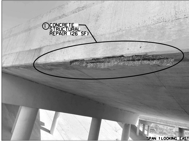
SPAN 1 LOOKING EAST
