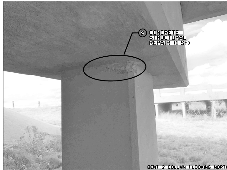
BENT 2 COLUMN 1 LOOKING NORTH
