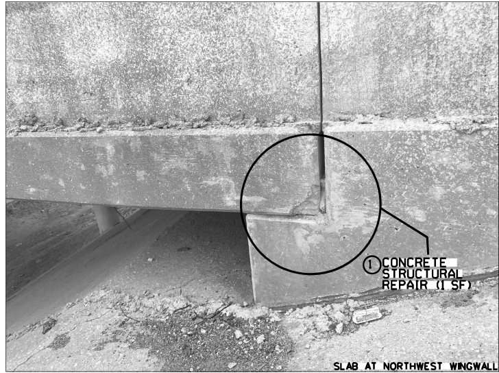
SLAB AT NORTHWEST WINGWALL
