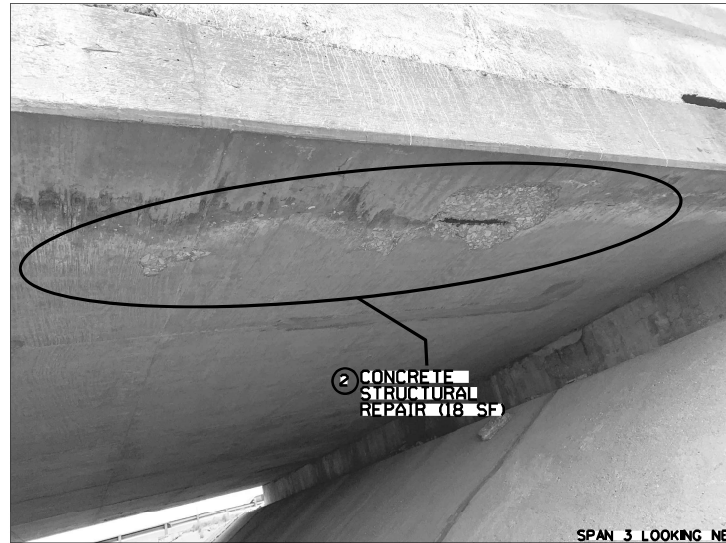
SPAN 3 LOOKING NE
