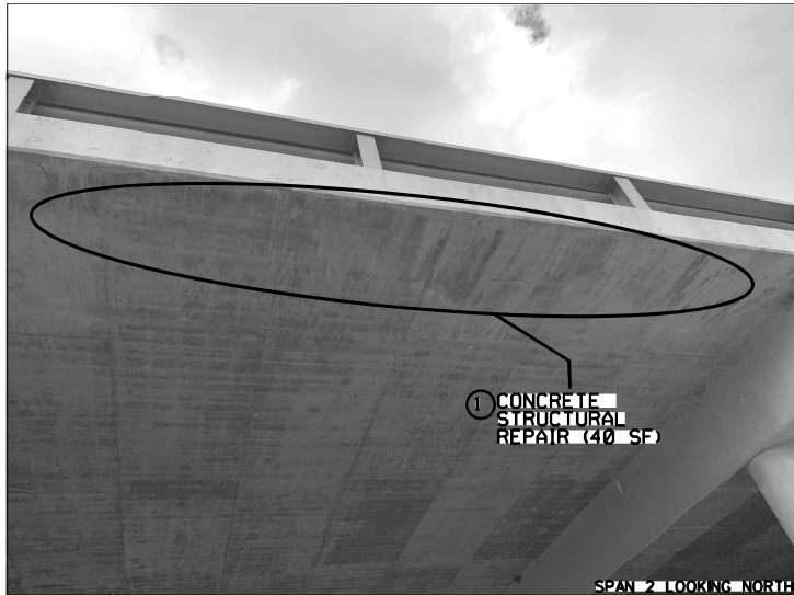
SPAN 2 LOOKING NORTH
