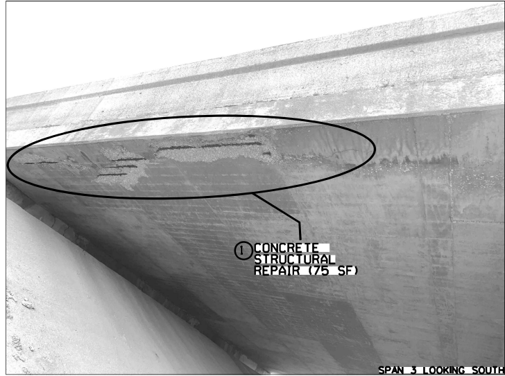
SPAN 3 LOOKING SOUTH
