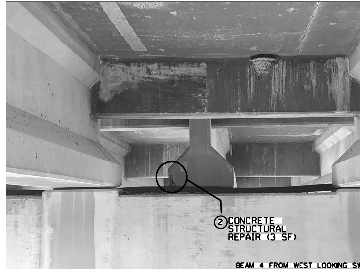
BEAM 4 FROM WEST LOOKING SW
