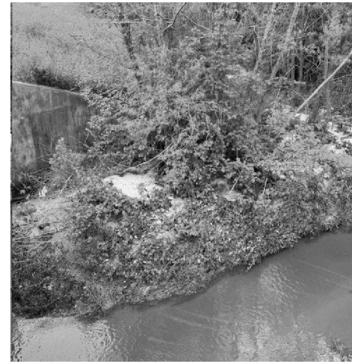
TYPICAL EROSION (M2) PHOTOS
