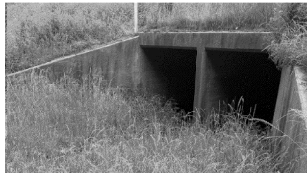
TYPICAL BENT (SBI) PHOTOS
