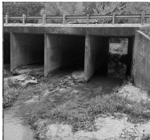
TYPICAL BENT (SBI) PHOTOS
