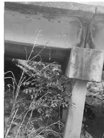
TYPICAL BENT (SBI) PHOTOS
