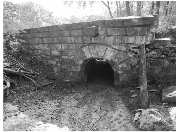
EXISTING CONDITIONS IMAGE. STA. 41+10 36" x 24' CMP
