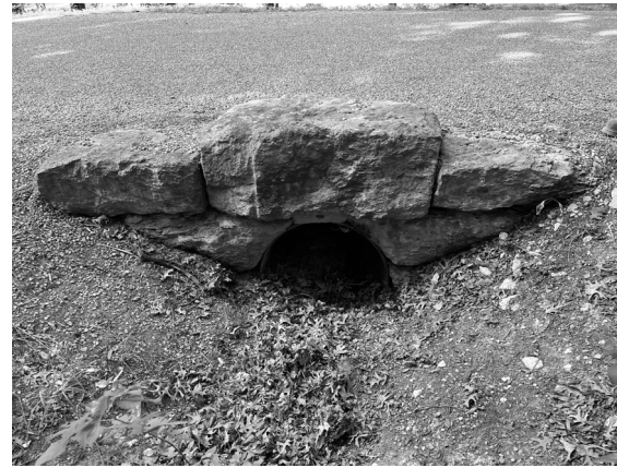
EXISTING CONDITIONS IMAGE. STA. 49+69 24" x 20' CMP
