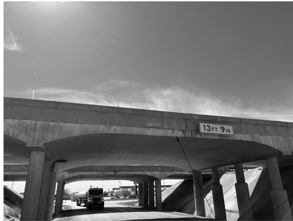
Repair fascia, install carbon fiber protection wrap
