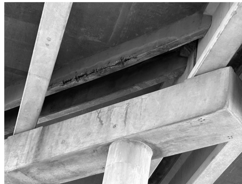
④ DIAPHRAGM REPAIR
