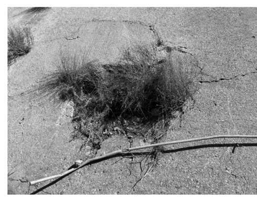
① CONCRETE RIPRAP REPAIR
