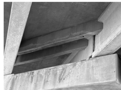
③ BENT CAP REPAIR
