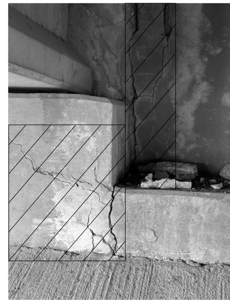
② PATCH ABUTMENT 11 NW WIDENING JOINT AND BACKWALL
