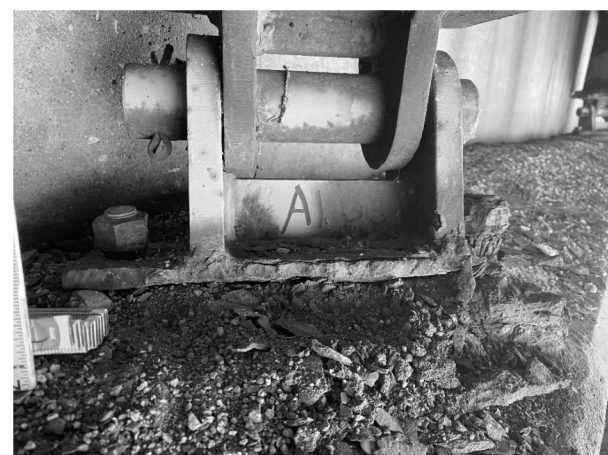
TYPICAL EXISTING BEARING
