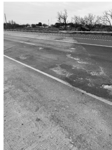
① APPROACH SLAB TYPICAL CONDITION
