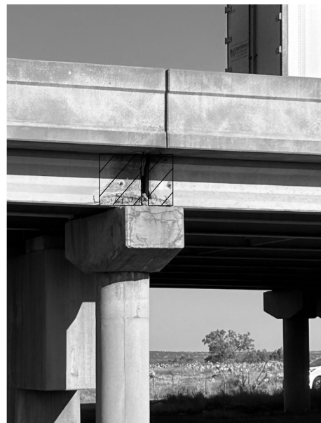
③ REPAIR SOUTH FASCIA BEAMS AT BENT 9
