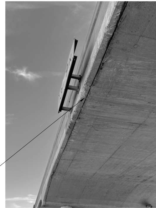
Repair fascia, install carbon fiber protection wrap
