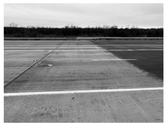
① APPROACH SLAB TYPICAL CONDITION
