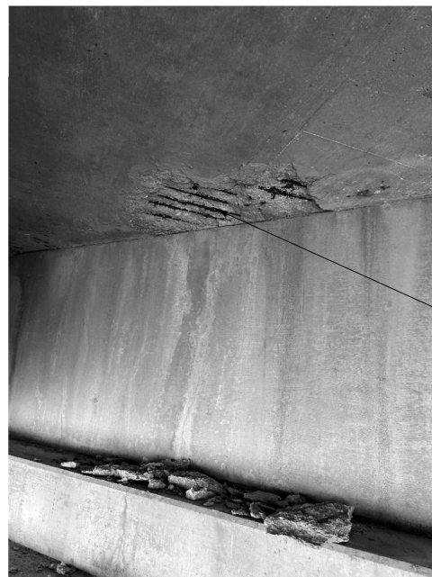
② DECK SOFFIT DELAMINATION
