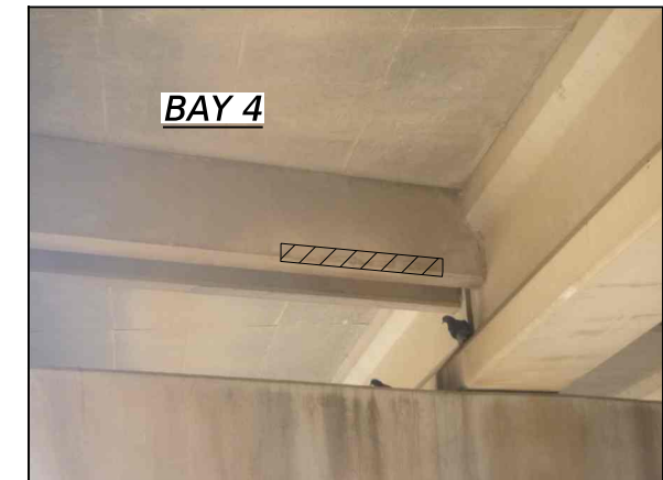
⑤ CONCRETE DIAPHRAGM REPAIR
