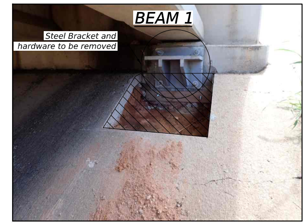
⑫ STEEL BRACKET REMOVAL
