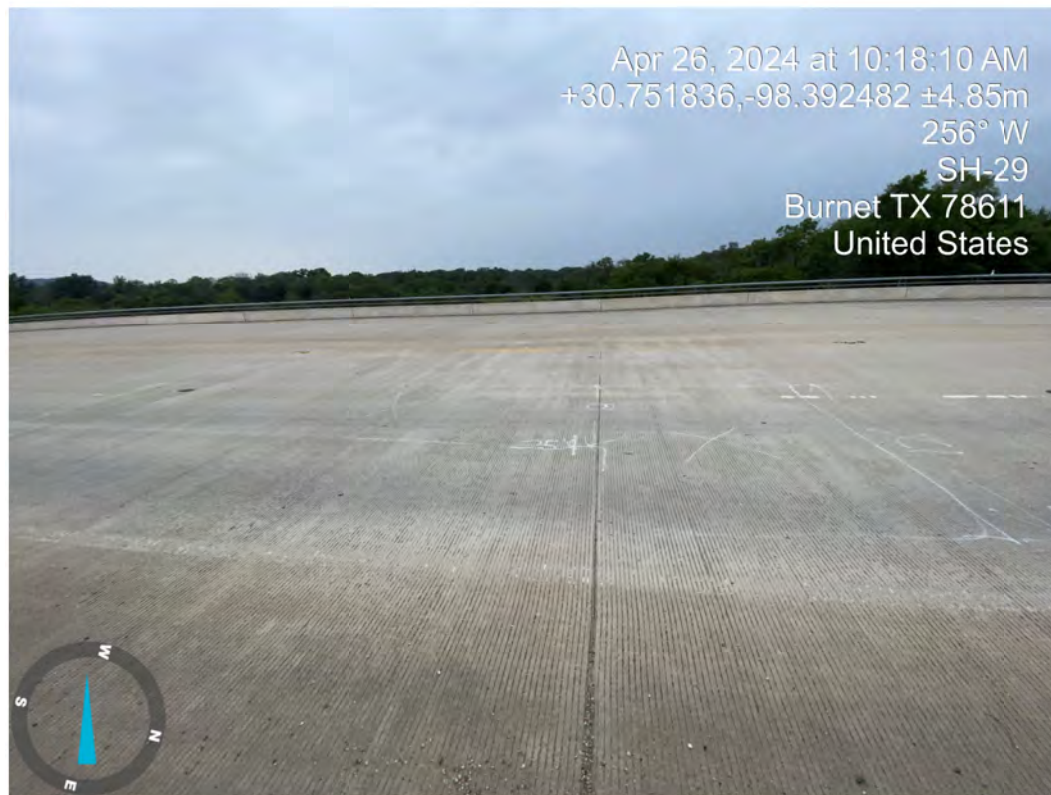
PHOTO 3: SPAN 3-4 - EASTBOUND LANES
