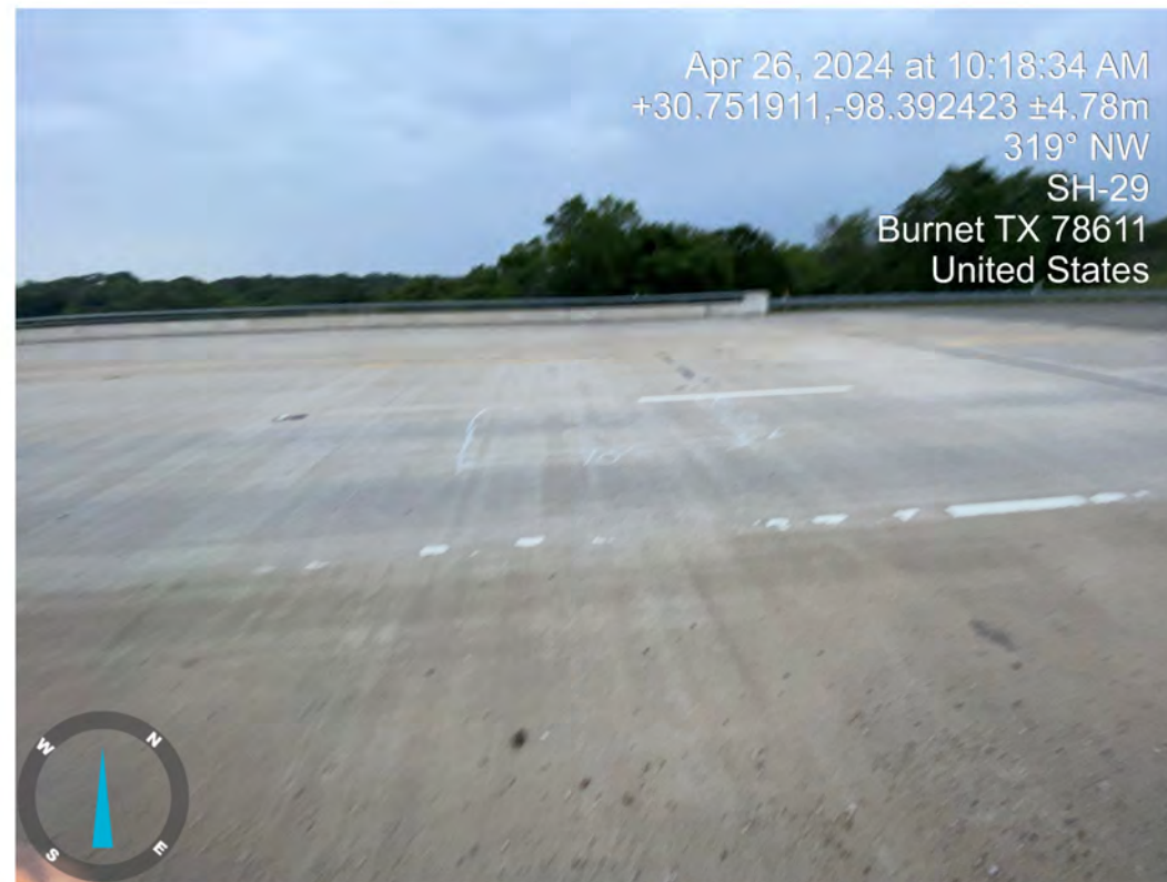
PHOTO 4: SPAN 4 - EASTBOUND LANES
