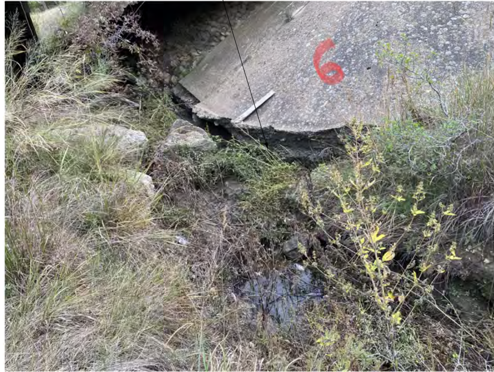
SOUTHWEST CORNER ABUTMENT 1
