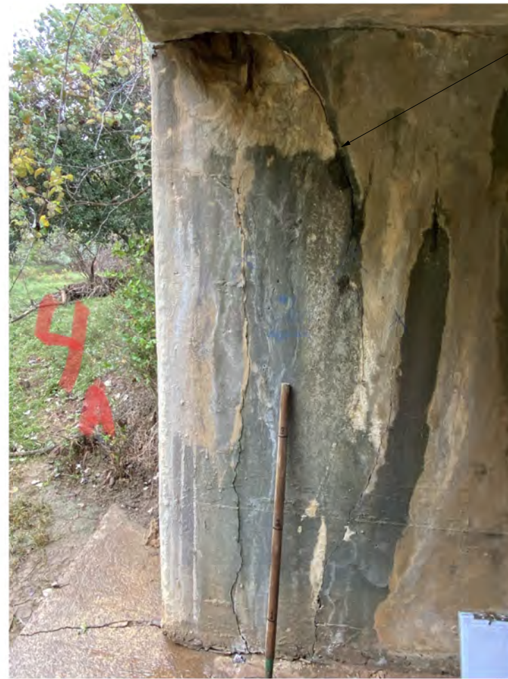
NORTH ABUTMENT WALL
