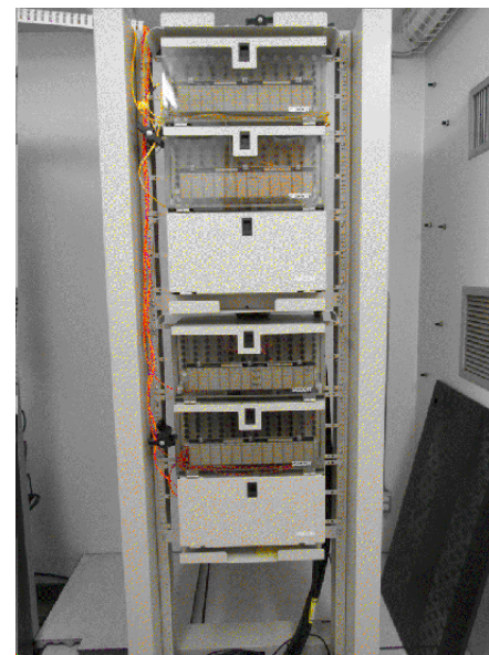
FIBER PATCH PANEL UNIT, PATCH PANELS, AND SPLICE ENCLOSURE (CORNING)
