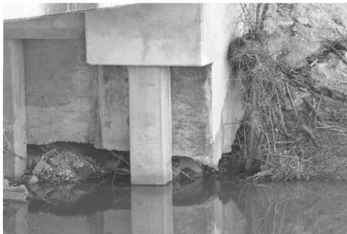
BROKEN RIPRAP AT NORTH CORNER
