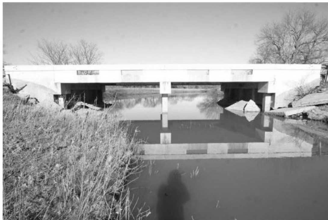
STREAM UNDER BRIDGE
