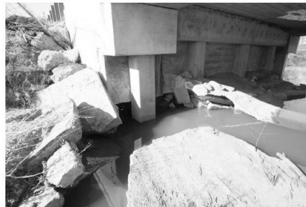
BROKEN RIPRAP AT WEST CORNER
