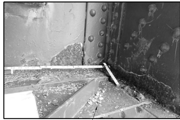
Replace connection plate
