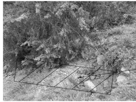
23 feet long by 4 feet wide by 3 feet deep washout as measured 9/30/2023. Fill with stone.
