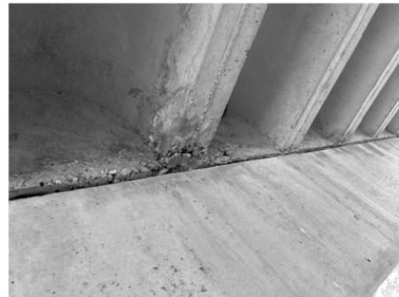
① CRACKING AND SPALLING IN DIAPHRAGMS 7N AND 6N AT BENT 3
