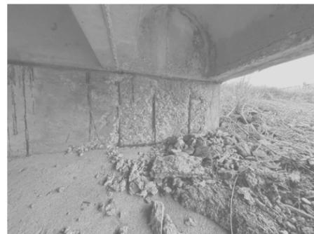
① DELAMINATION AND SPALLING SOUTHEAST QUADRANT OF ABUTMENT 5
