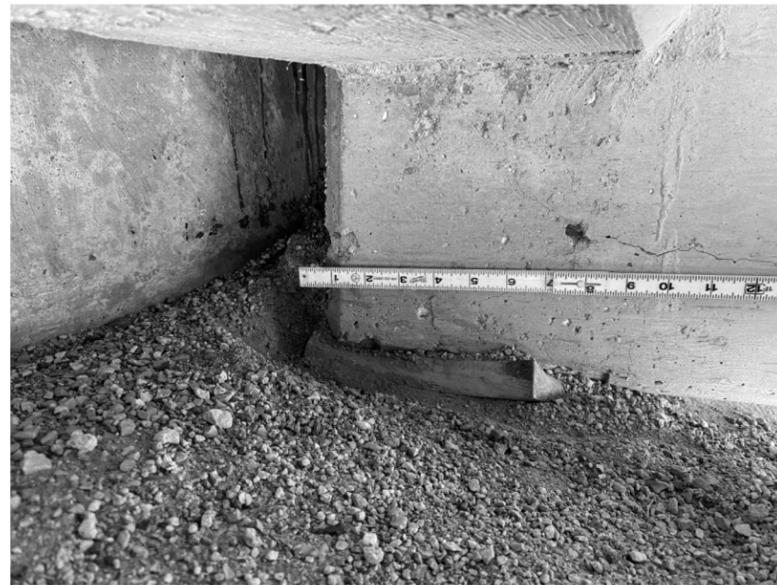
**① REPLACE ELASTOMERIC PADS AND CLEAN ABUTMENT TOPS - TYPICAL**
