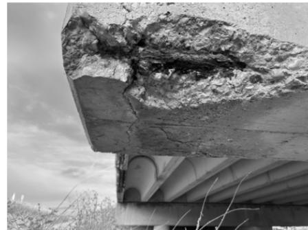
① CRACKING AND SPALLING ON THE BOTTOM OF SOUTH OVERHANG OF BENT 3
