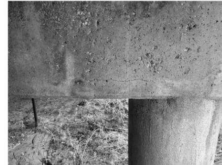
① BOTTOM OF CAP CRACKING AT WEST FACE OF BENT 2
