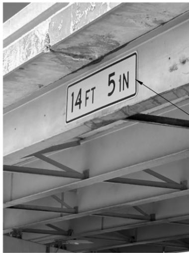
Remove and salvage clearance sign prior to heat straightening and re-install after painting. This work is subsidiary to heat straightening.
