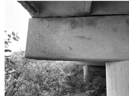
① CRACKING AND DELAMINATION ON THE BOTTOM OF NORTH OVERHANG OF BENT 3
