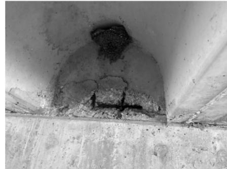
① CRACKING AND SPALLING IN BAY 7N DIAPHRAGM AT BENT 2
