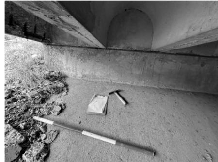
① DELAMINATION AND CRACKING AT ABUTMENT 1 UNDER BEAM 14N AND BETWEEN BEAMS 12N AND 13N
