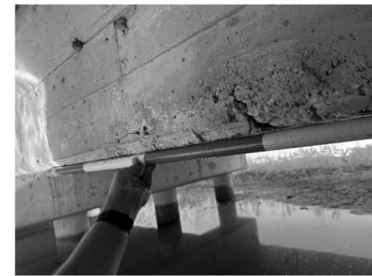
**① CRACKING AND DELAMINATION AT BOTTOM OF STEM ON BEAM 5W, SPAN 3**
