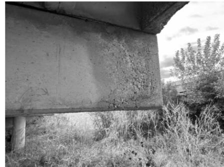
③ CRACKING AND DELAMINATION ON BOTTOM OF WEST FACE OF SOUTH OVERHANG OF BENT 3
