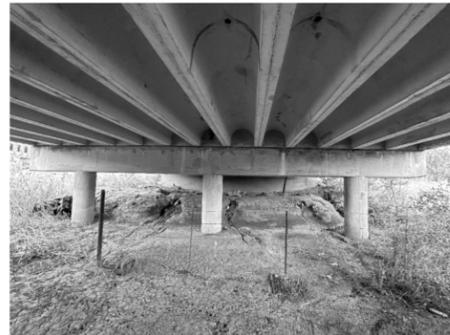
① EAST FACE BENT 2W SHOWING DELAMINATION IN DIAPHRAGM IN BAY 7N
