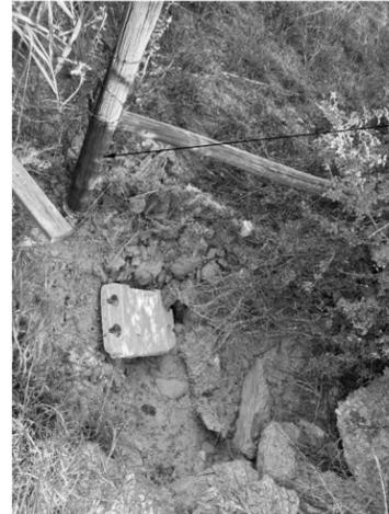
Remove and replace wire fence located within washout repair as directed by the Engineer, to facilitate placement of stone protection.
