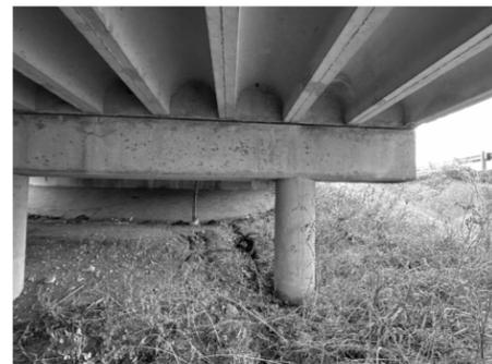
① DELAMINATION ON WEST FACE BENT 4 UNDER BEAMS 9N, 12N, 13N, AND 14N
