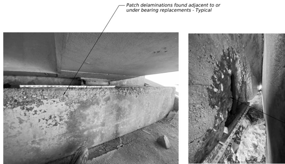
Patch delaminations found adjacent to or under bearing replacements - Typical
