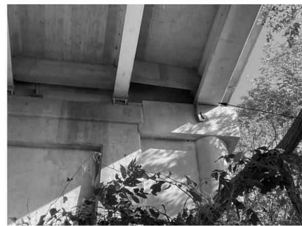
Replace Elastomeric Bearing Pads on Concrete Exterior Fascia Beams at the locations shown on the Plans. Existing Elastomeric Bearing Plans are not available. Verify all field dimension prior to fabrication of bearing pads.
