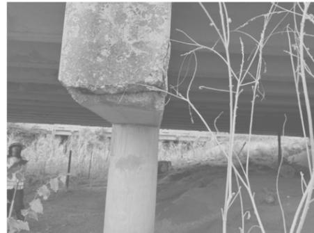
① SPALLING IN NORTH CANTILEVER OF BENT 2 ON NORTH SIDE
