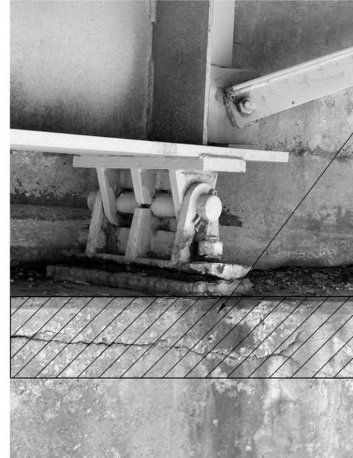
Patch delaminations found adjacent to or under bearing replacements (Typical)
