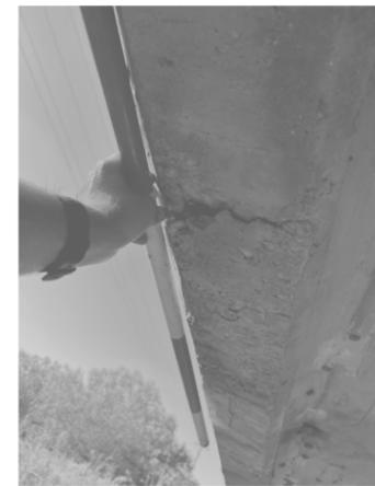
**① CRACKING AND DELAMINATION AT BOTTOM OF STEM ON BEAM 1W, SPAN 3**
