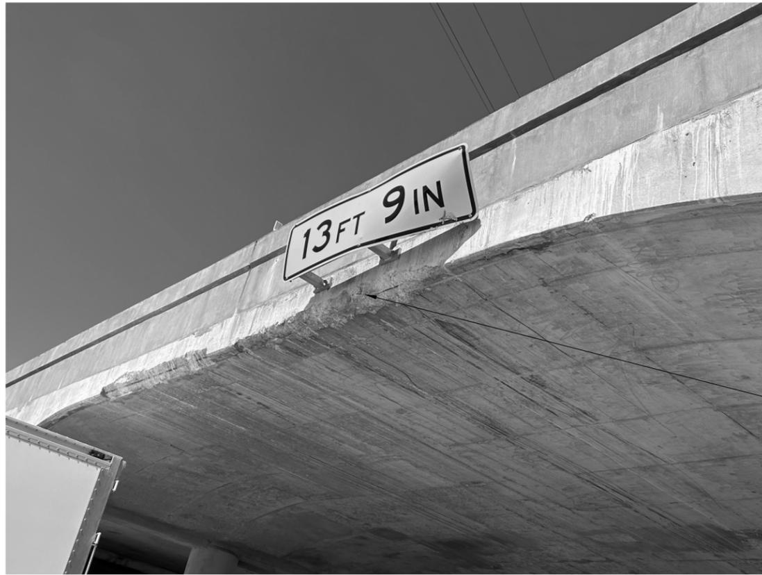
Remove clearance sign, repair fascia, install carbon fiber protection wrap and install new clearance sign.
