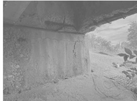
① DELAMINATION AND SPALLING IN NORTHWEST QUADRANT OF ABUTMENT 1 AND DIAPHRAGM OF BAY 1N
