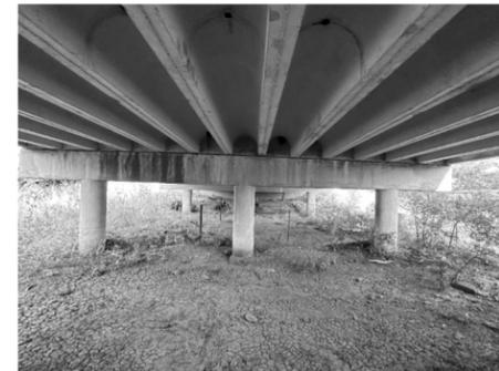
① EAST FACE BENT 3 SHOWING 3FT OF CORNER CRACKING ON BOTTOM OF BENT 2 NORTH CANTILEVER
