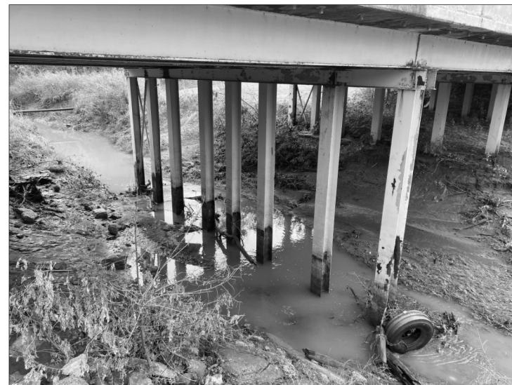
TYPICAL PILES FOR ENCASEMENT (SB1)
