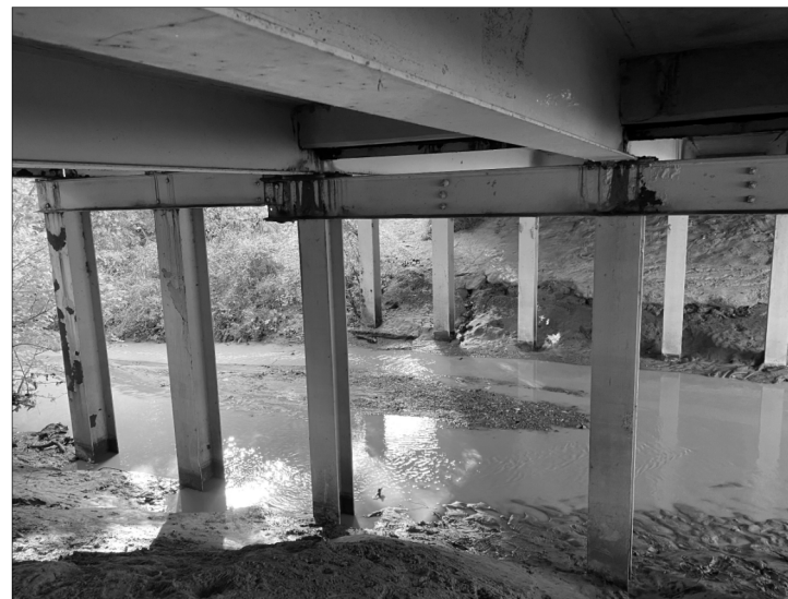
TYPICAL STEEL PAINTING ON BEAMS, BENT CAPS AND PILING (SP1)
