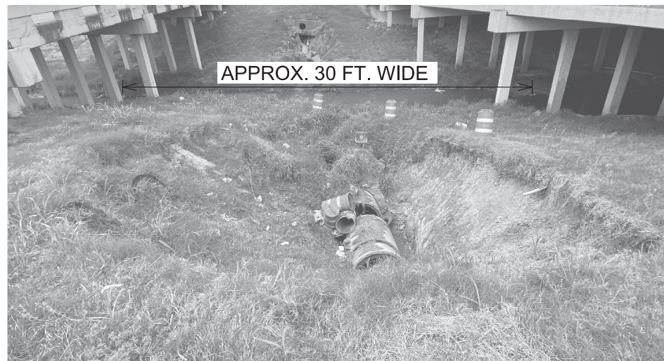
DOWNHILL VIEW OF OUTFALL DAMAGE (Photo taken on 3-08-2023)
