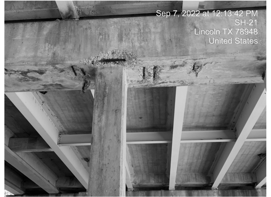
More exposed reinforcement is common through out the bridge.
