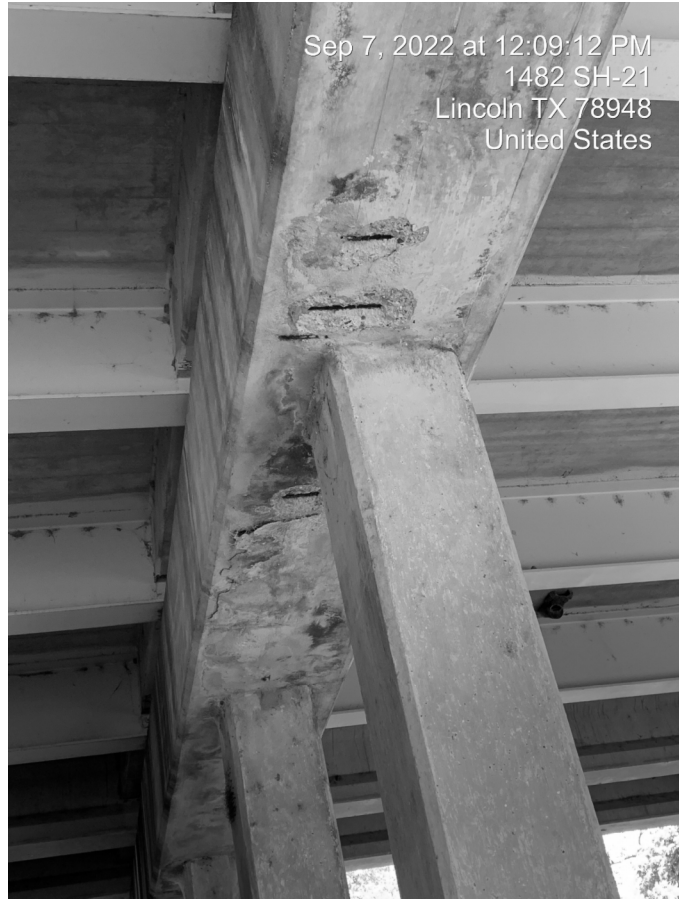
Exposed reinforcement at bent cap.
