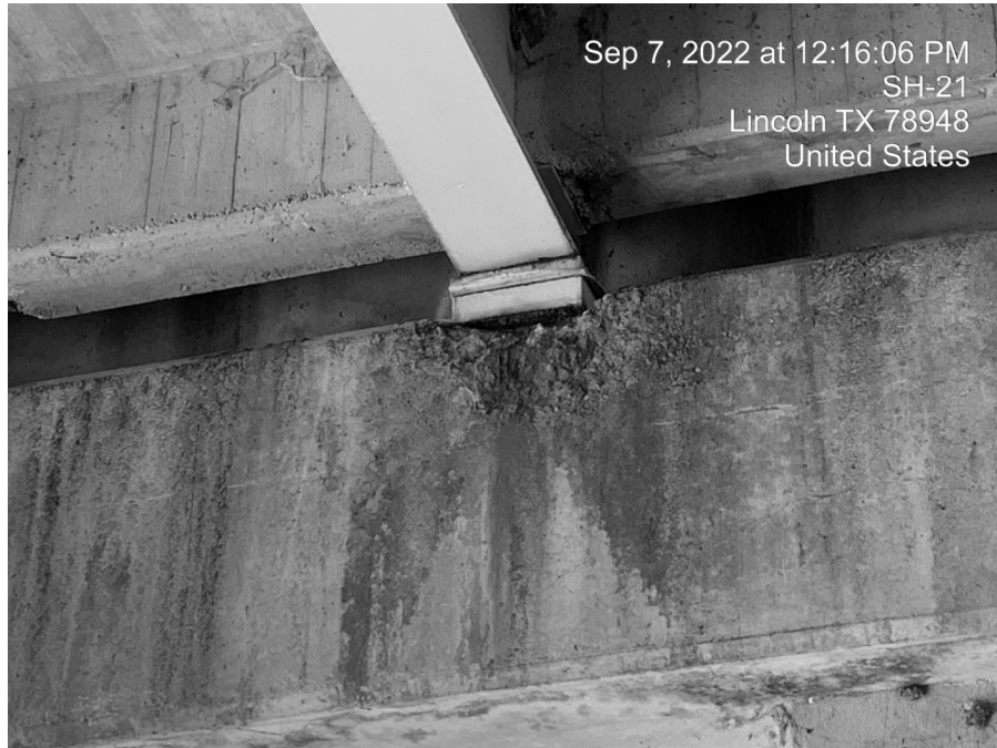
Concrete loss under bearing pad.
