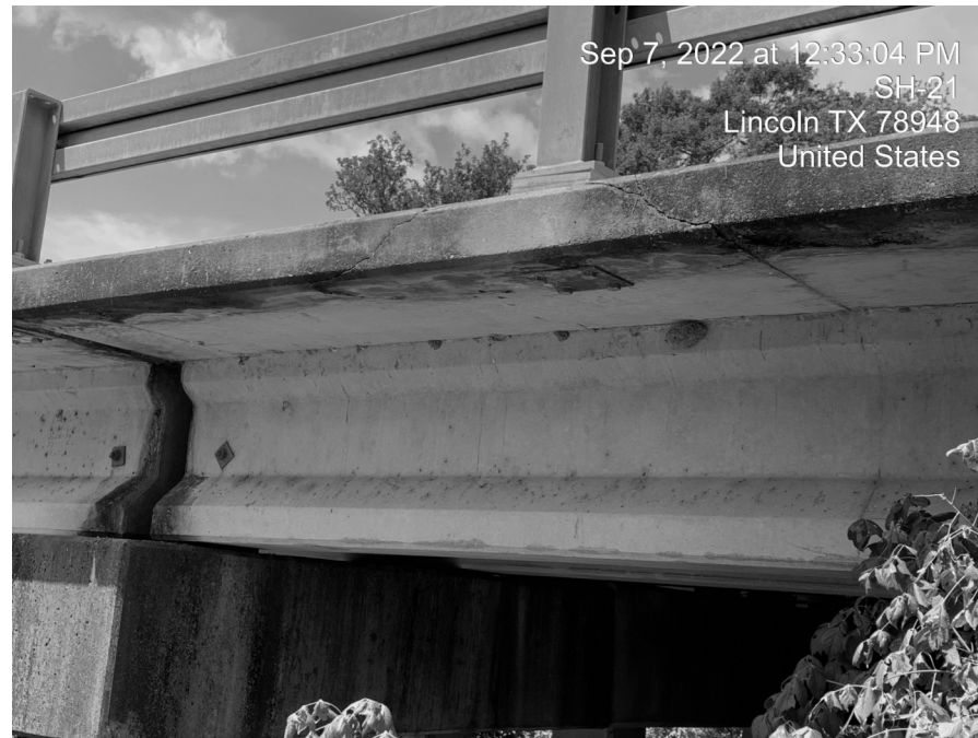
Cracks under post of existing bridge rail.
