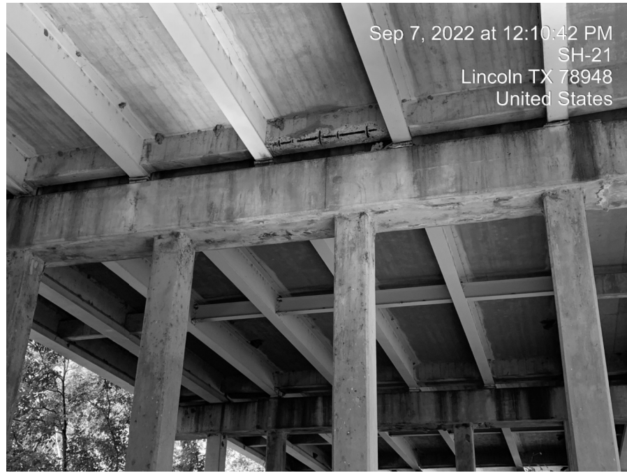
Exposed reinforcement on diaphragm.
