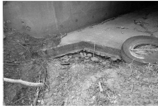
DOWNSTREAM TOE WALL
