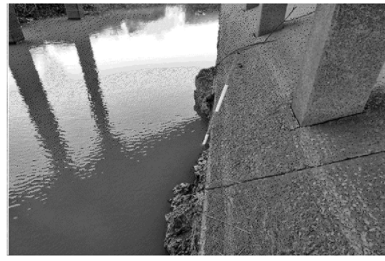
EAST TOEWALL EXPOSED
