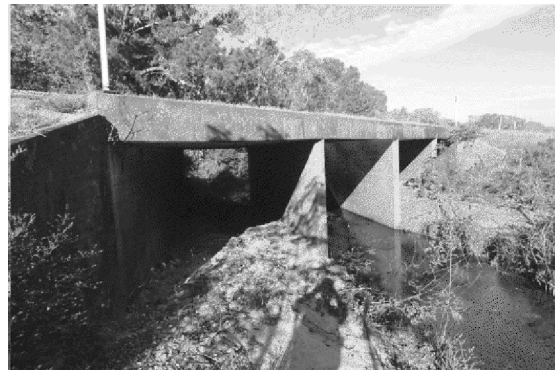
ELEVATION LOOKING WEST
