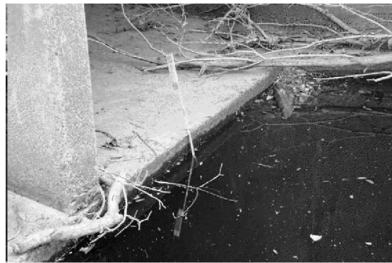
UPSTREAM TOE WALL
