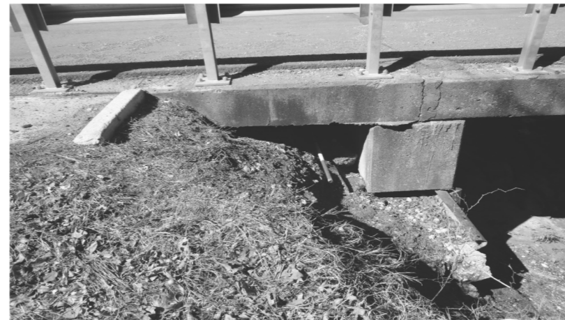
SOUTHEAST END OF SOUTHWEST ABUTMENT CAP LOOKING NORTHWEST
