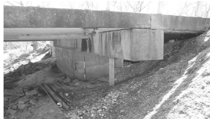
NORTHWEST END OF SOUTHWEST ABUTMENT CAP LOOKING NORTHWEST
