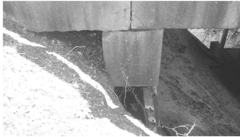
NORTHWEST END OF NORTHEAST ABUTMENT CAP LOOKING SOUTHEAST
