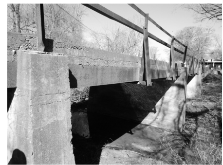
Three Interior Bents
