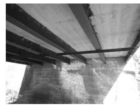
View of Interior Bent and Superstructure from below
