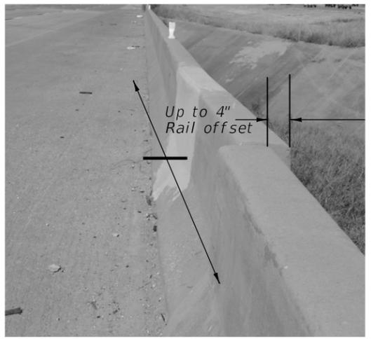
Bridge rail has laterally moved due to impact damage.
