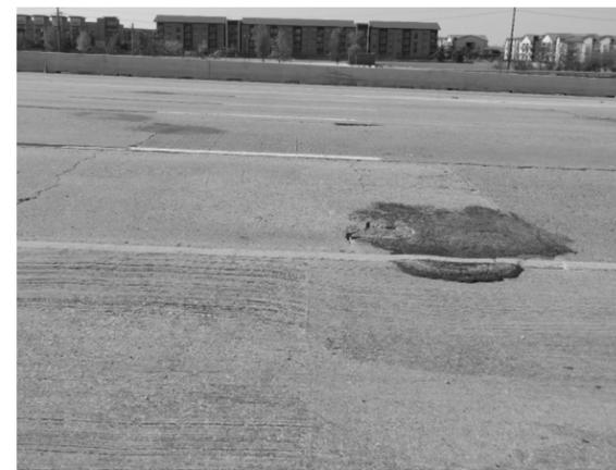
D4: Cracks, spalls, and settlement at NW corner of approach slab.
