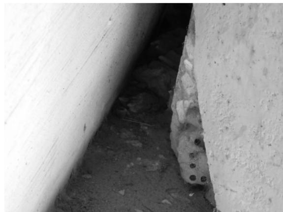
SP1: Spall on beam end at east abutment (TYP).
