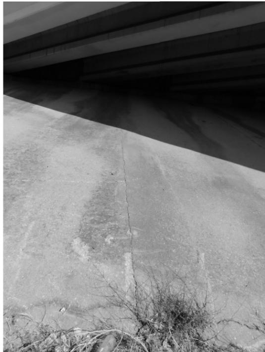
M2: Cracks at SW corner of concrete riprap at west abutment.
