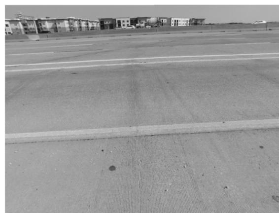
D5: Cracks at deck surface.
