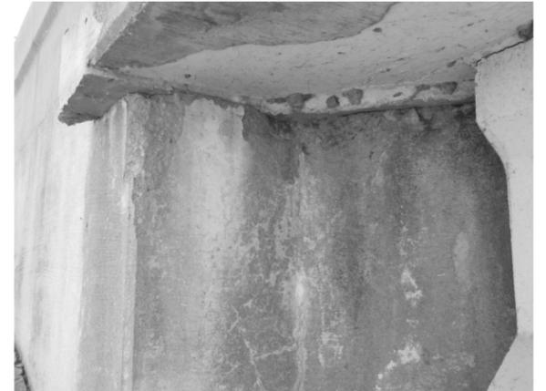
SB1: Concrete spall at east abutment backwall (NE corner).
