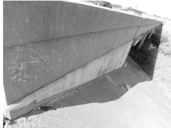
M1: Separation of concrete riprap and wingwall at west abutment.
