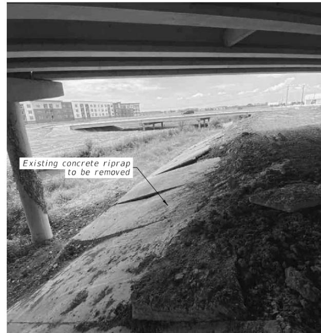
③ Looking North at broken concrete riprap to be removed and replaced
