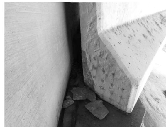
SP1: Spall on beam end at west abutment (TYP).
