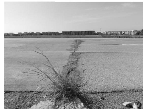
D2a/ D2b/ D2c: Cracks, spalls, and vegetation along the relief joint.
