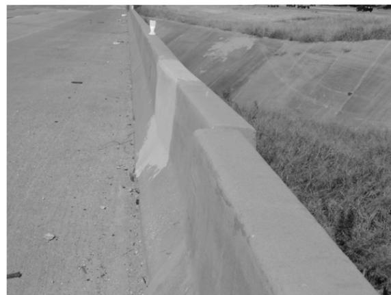
R2: Bridge rail has laterally moved due to impact damage.
