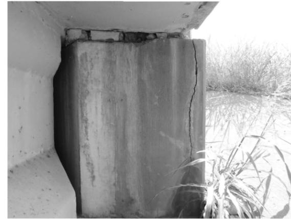
SB1: Delamination at east abutment backwall (SE corner).
