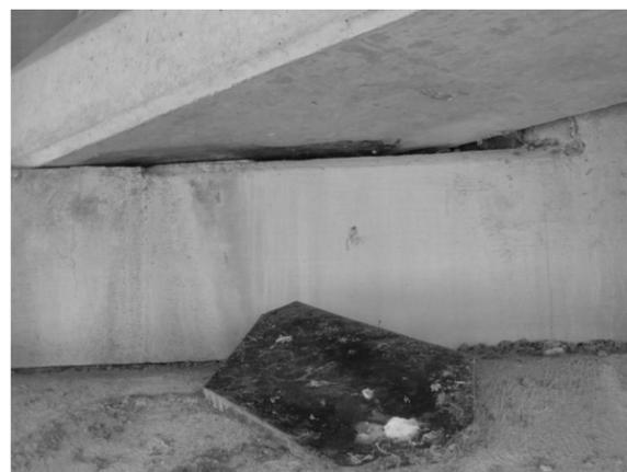
SP2: Missing elastomeric bearing pad at both abutment (TYP).
