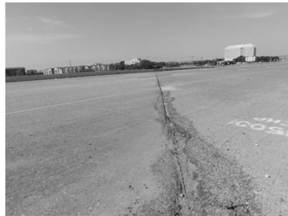
D1a/ D1b/ D1c/R1: Joint seals along abutments are torn with minor spalls.
