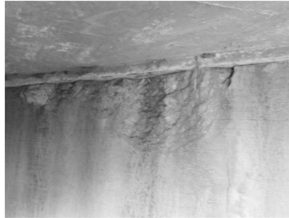
SB1: Moderate spall at west abutment backwall.
