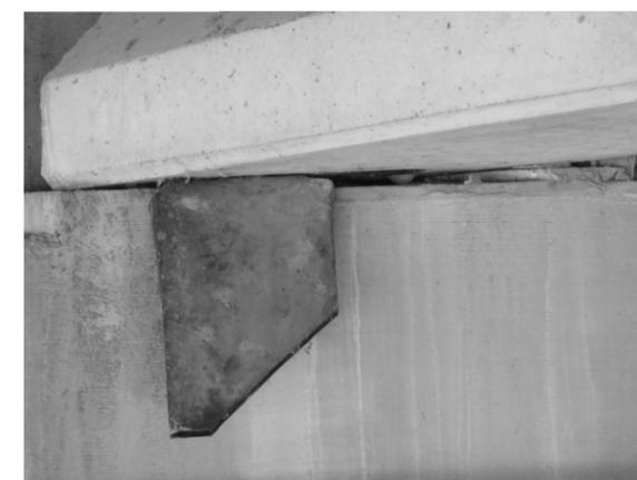
SP2: Slipped elastomeric bearing pad at both abutment (TYP).
