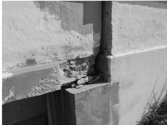
D6: Moderate spall with exposed rebar at deck overhang.
