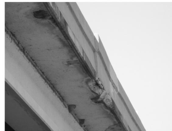
D3: Spall with exposed rebar along north edge of deck of span 2 from west.
