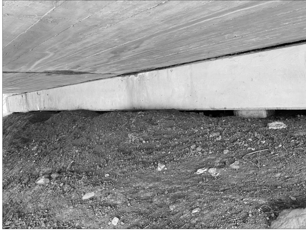
ABUTMENT UNDERMINING
