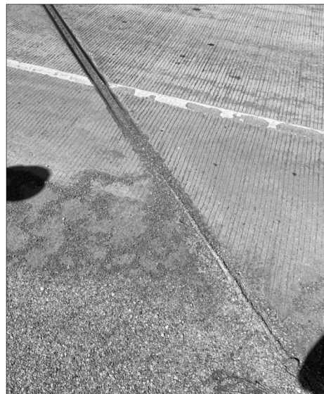
TYPICAL DEBRIS COMPACTION IN JOINTS
