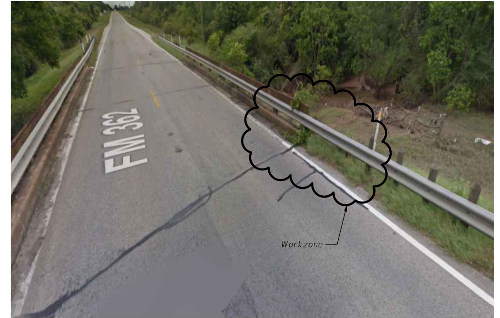
SOUTHEAST WINGWALL PHOTO Looking North
