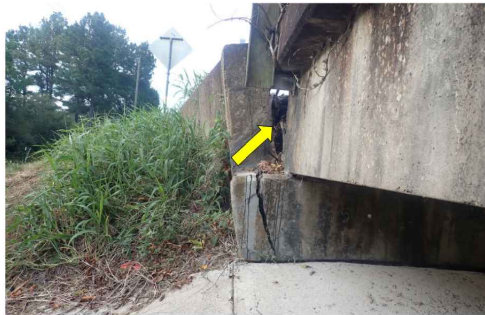
SOUTHEAST WINGWALL PHOTO Looking South ~ August 2020
