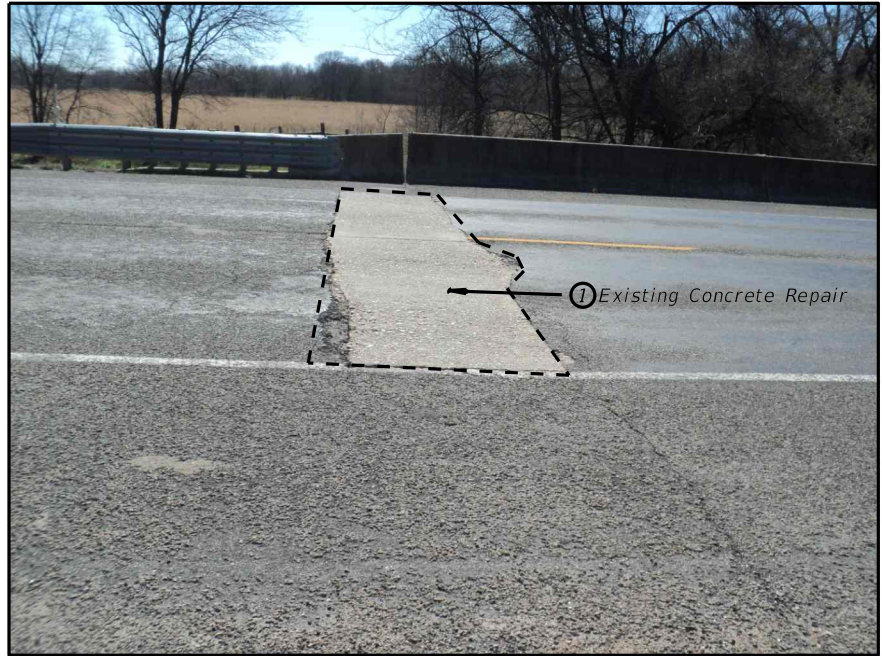
EXISTING CONCRETE REPAIR AT END OF BRIDGE (REPAIR LOCATION B)
