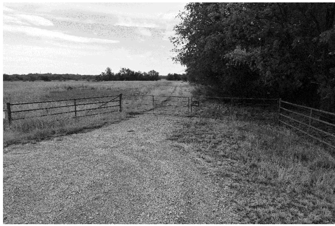
EXISTING DRIVEWAY 02 GATE CONSTRUCTION
