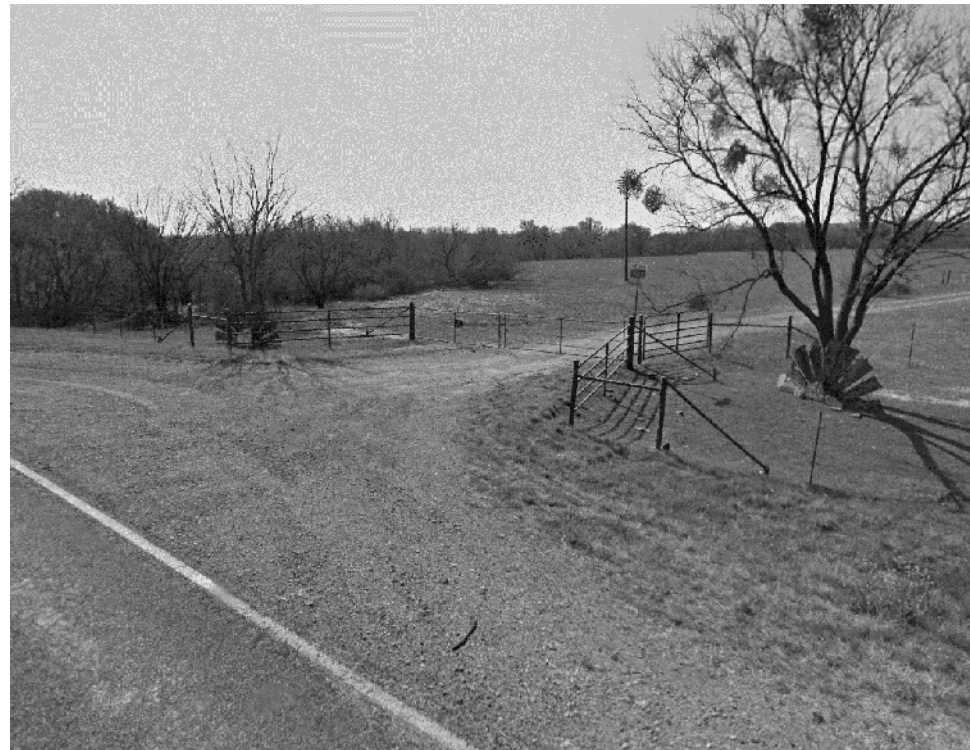
EXISTING DRIVEWAY 01 GATE CONSTRUCTION
