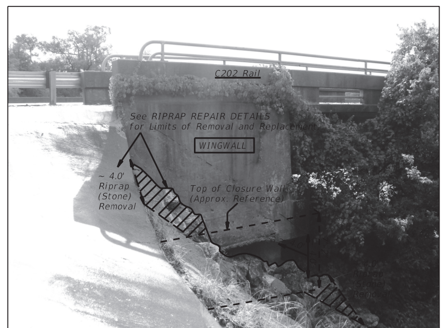
★ EROSION REPAIR AT WINGWALL (SHOWING LIMITS OF REPAIR) (LOOKING EAST)
