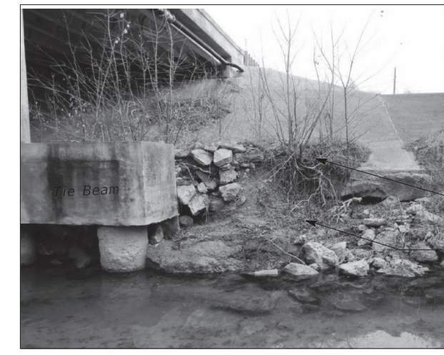
② REPAIR AT EXISTING RIPRAP TOEWALL SHOWING LIMITS OF REPAIR AREA UPSTREAM SOUTH BANKS
