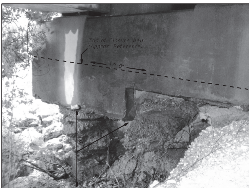
★ EROSION REPAIR AT ABUTMENT #5 (SHOWING LIMITS OF REPAIR) (LOOKING NORTHWEST)
