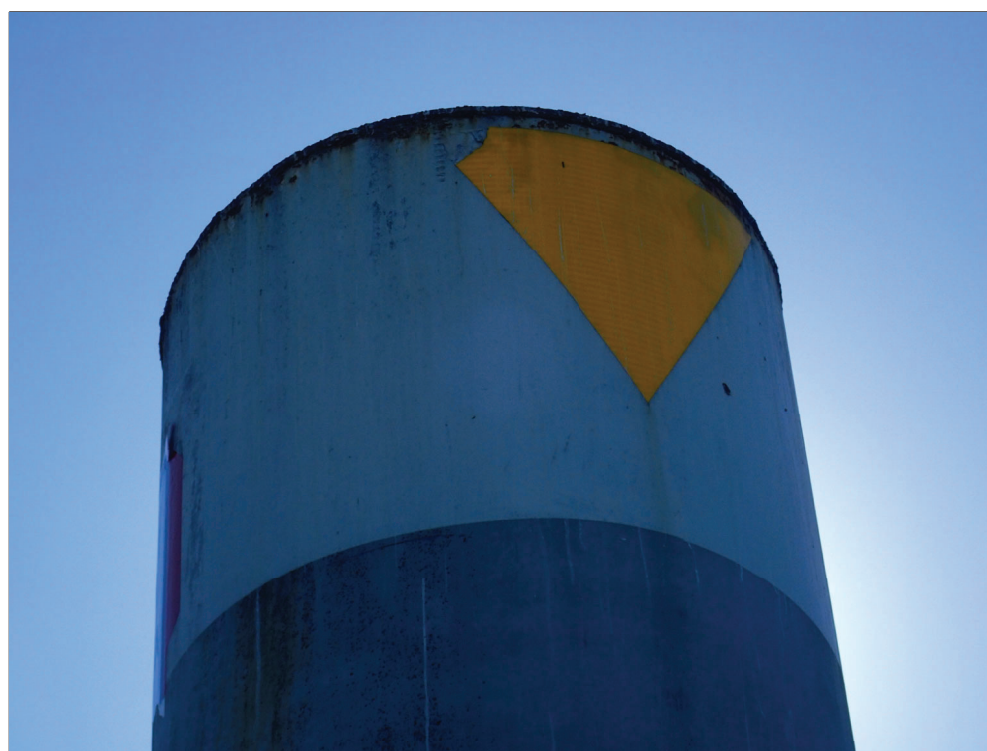
RETRO-REFLECTIVE ADHESIVE SIGN ON INTERMEDIATE DOLPHIN (TRIANGLE)
