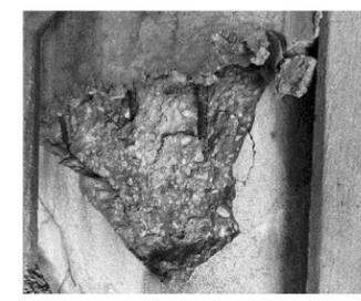
48"x48"x5" DEEP SPALL WITH EXPOSED REBAR AT ABUT 4 RIGHT OF BEAM 16.
