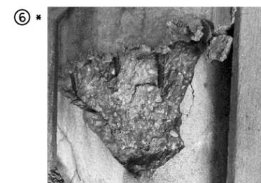
48"x48"x5" DEEP SPALL WITH EXPOSED REBAR AT ABUT 4 RIGHT OF BEAM 16.
