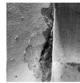
24"x48"x4" DEEP SPALL WITH EXPOSED REBAR AT ABUT 4 BEHIND BEAM 8.
