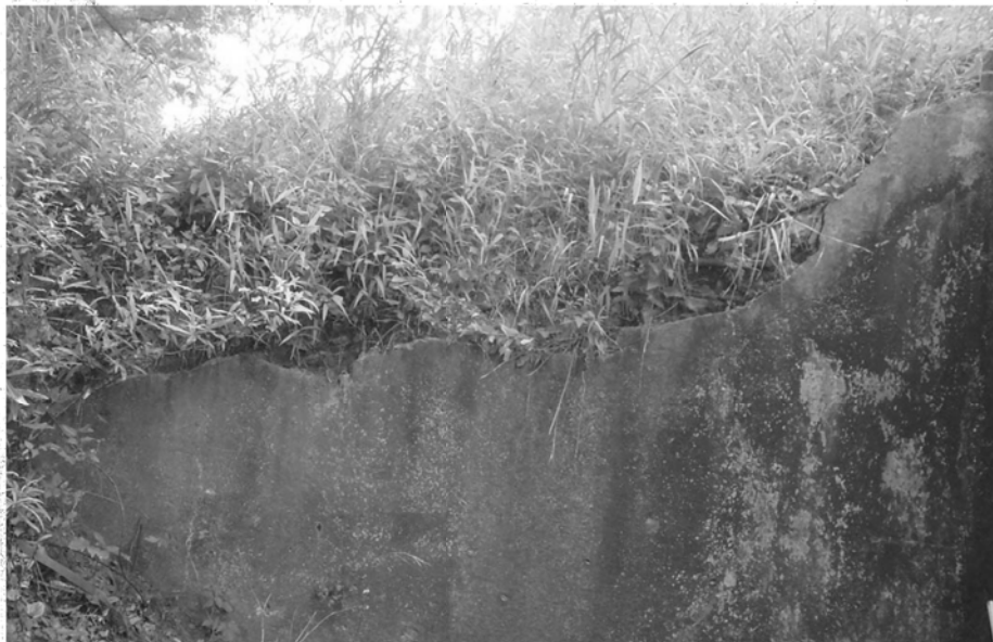
SPALLING AT SOUTHEAST WINGWALL
