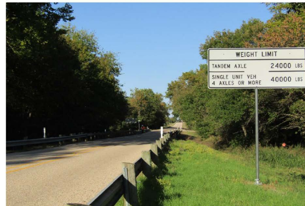
WEIGHT LIMIT SIGN AT SOUTHWEST END LOOKING NORTHEAST
