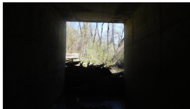
10 - Debris located in barrels
