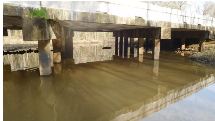
5 - Stream Under looking Northwest
