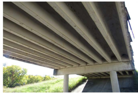
SUPERSTRUCTURE LOOKING SOUTHWEST
