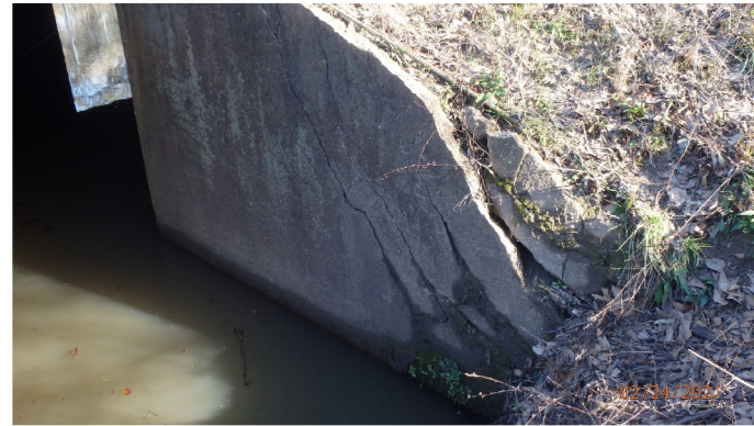
SOUTH WINGWALL LOOKING EAST
