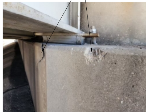
ABUTMENT 5 NORTH CORNER
