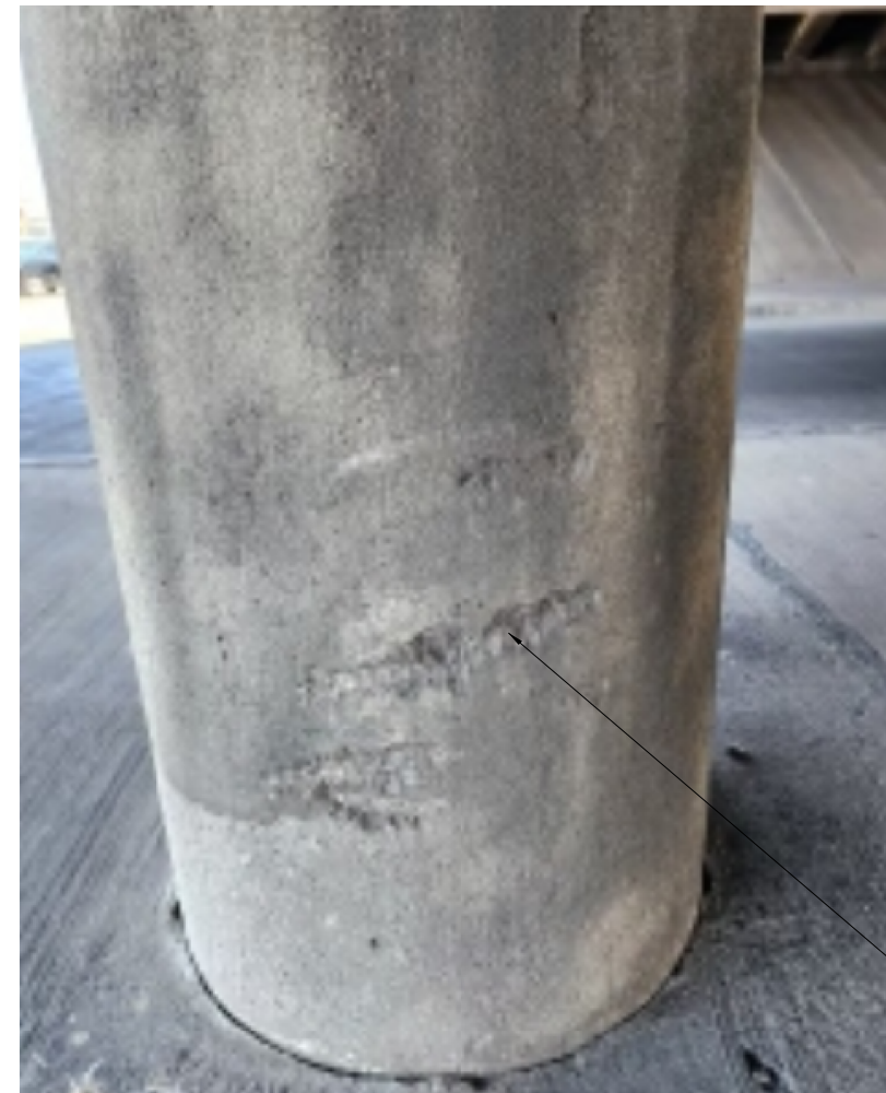
BENT 5 COLUMN 4 WEST FACE
