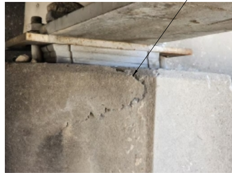
ABUTMENT 5 SOUTH CORNER
