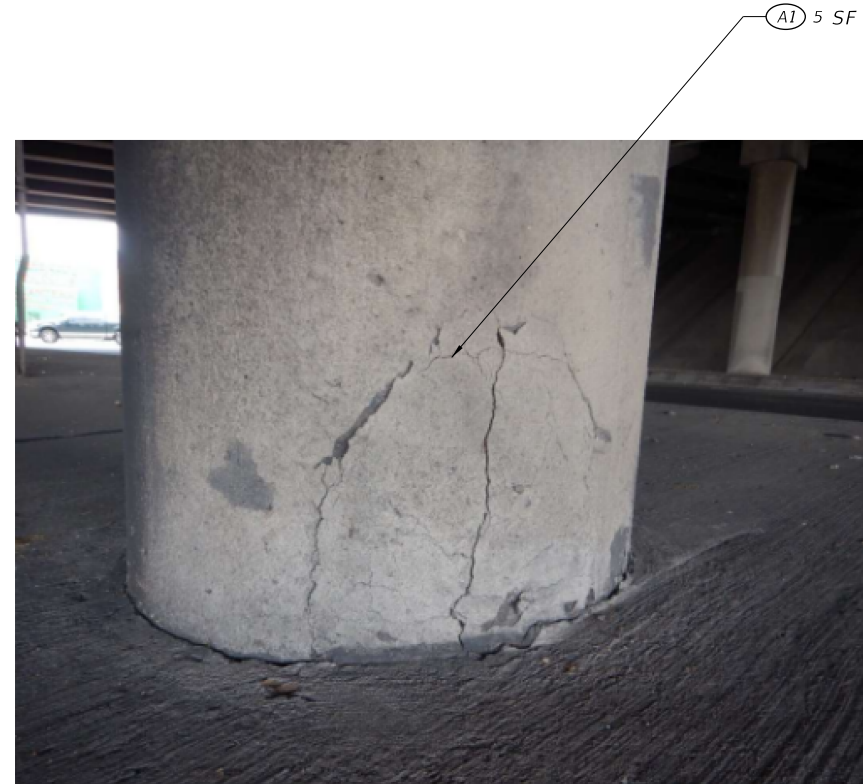
BENT 5 BASE OF COLUMN 3 SOUTH FACE
