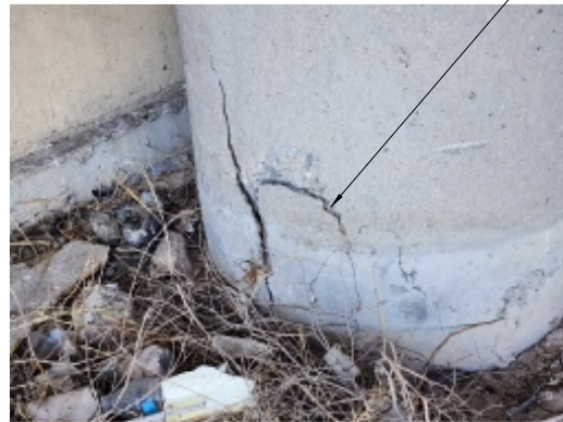
BENT 4 COLUMN 2 SOUTH FACE
