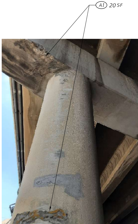
BENT 2 COLUMN 6 NORTH FACE
