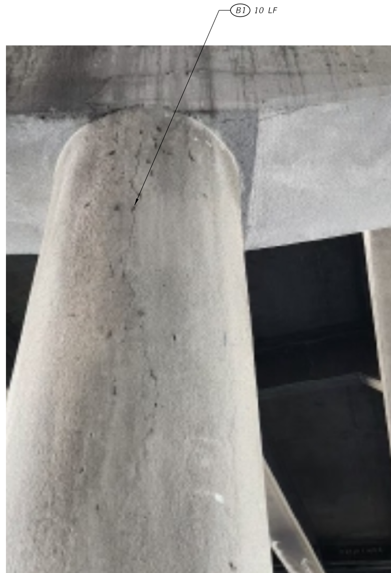
BENT 2 COLUMN 3 EAST FACE
