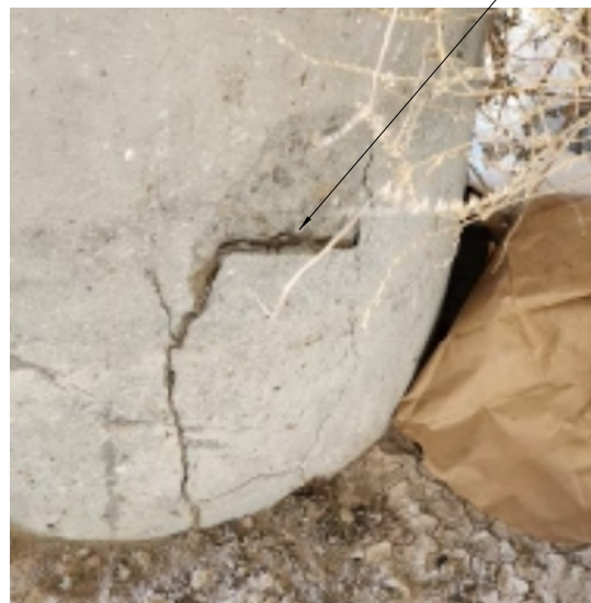
BENT 4 COLUMN 3 SOUTH FACE
