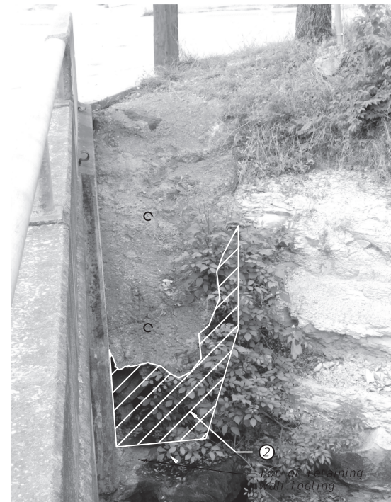
SW Bridge Corner
