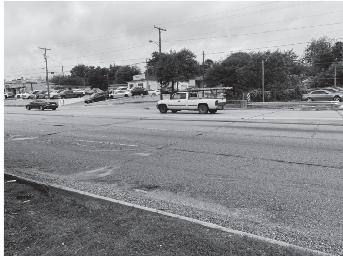
D1 - View of Bridge Deck from NE corner
