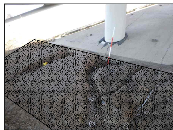
12 EXPOSED TOE RIPRAP TO BE COVERED WITH EMBANKMENT
