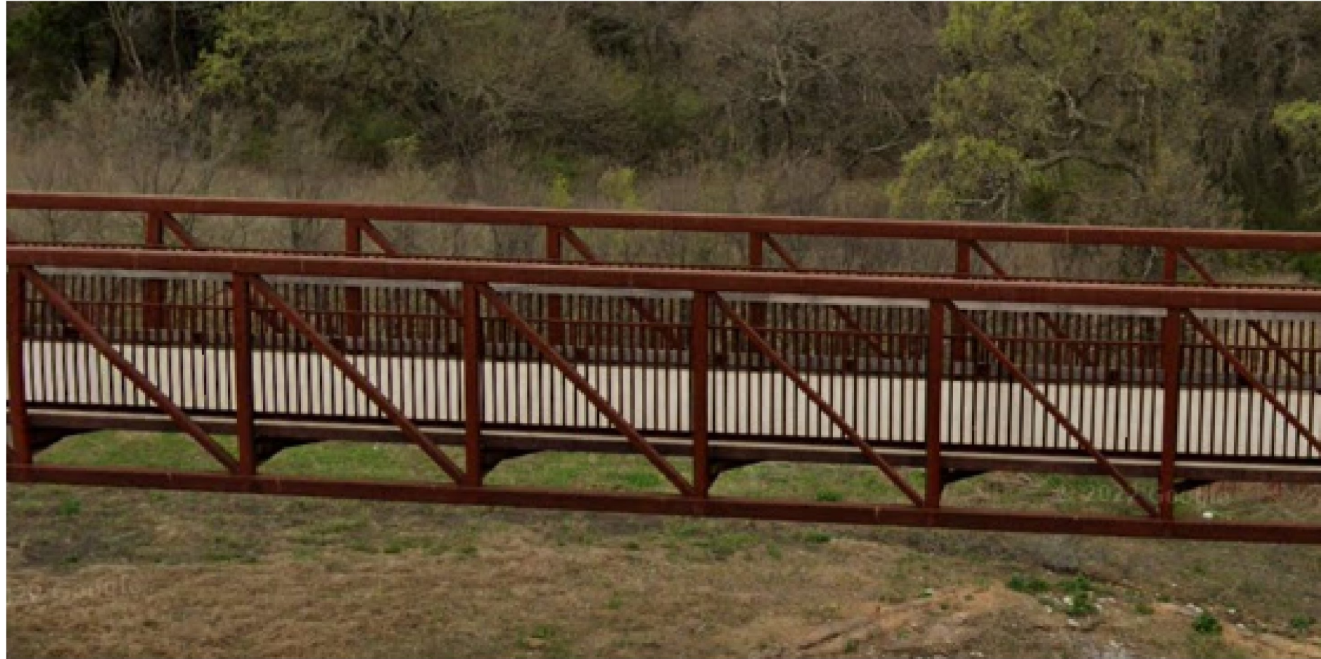
EXAMPLE BRIDGE (PEDESTRIAN BRIDGE ADJACENT TO FM 1382 IN CEDAR HILL, TEXAS)
