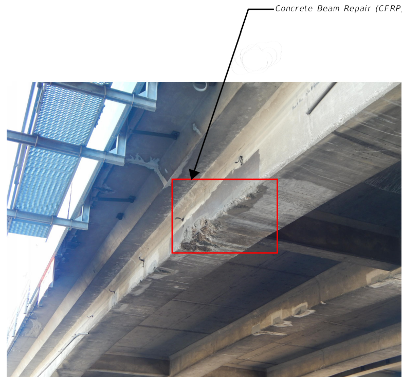
PHOTO 1 Span 3 Beam 1 (Looking Northeast)
