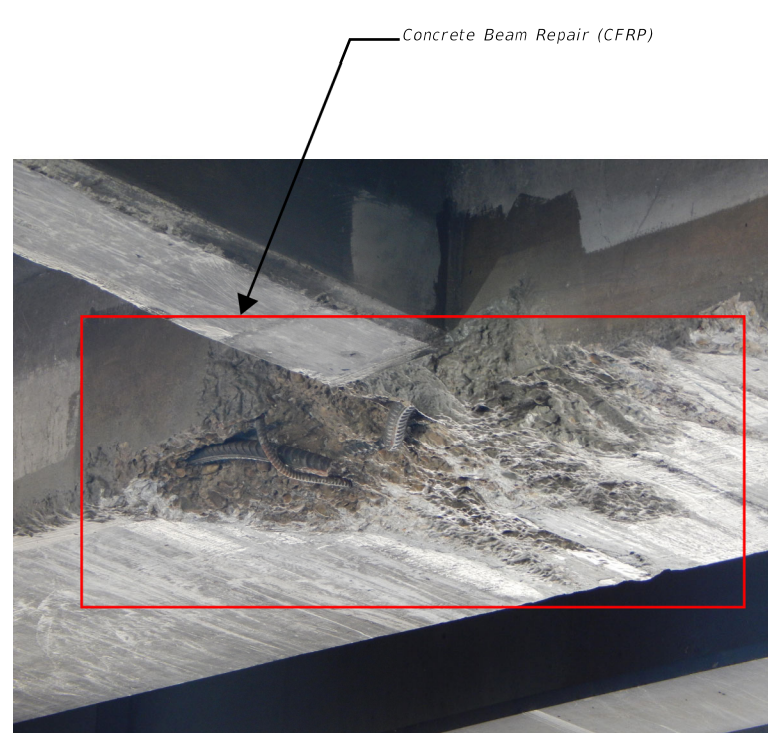
PHOTO 2 Span 3 Beam 3 (Looking Northeast)
