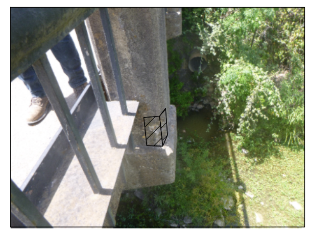
NE RAIL, 4TH POST FROM NORTH CORNER
