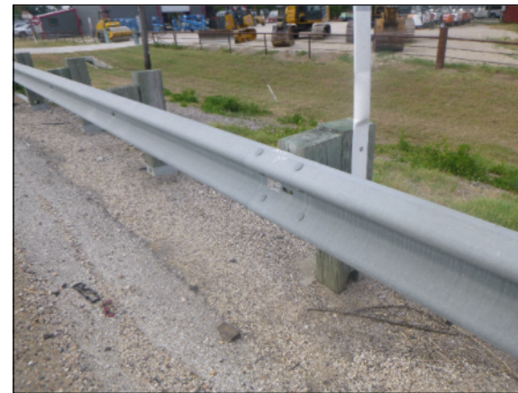
⑧ TYPICAL DISCONNECTED POST
