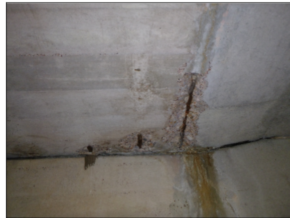
SPAN 5 SW WIDENING JOINT
