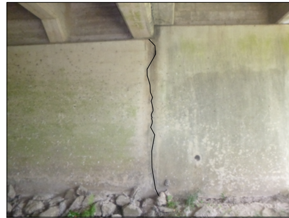
ABUTMENT 3, NE WIDENING JOINT (7) TYPICAL CRACK REPAIR
