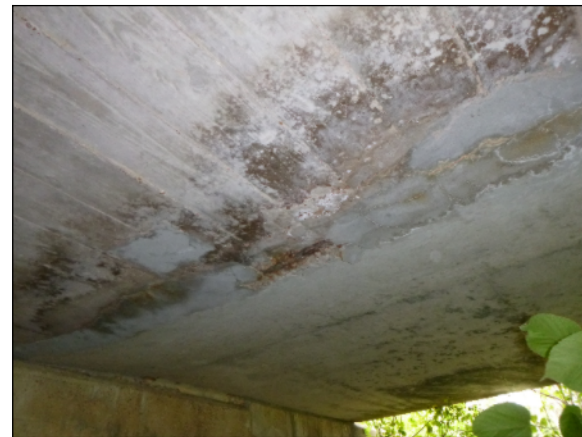
SPAN 1 SW WIDENING JOINT
