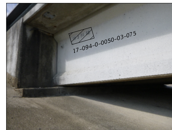
⑨ REMOVAL AND REPLACEMENT OF PAINTED NBI NUMBER
