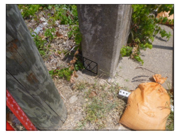
NE RAIL, POST AT NORTH CORNER
