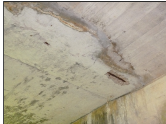
SPAN 2 NE WIDENING JOINT
