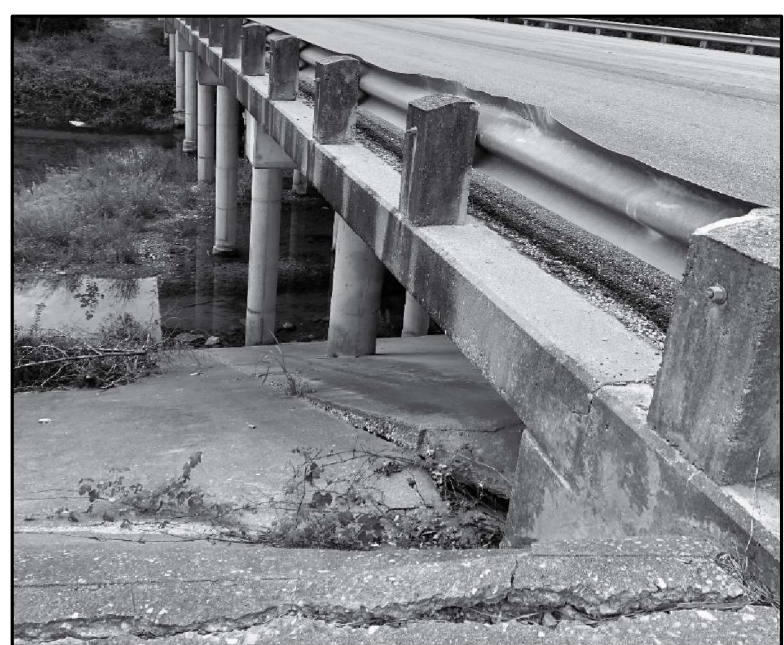
EXISTING CONCRETE RIPRAP, NE CORNER
