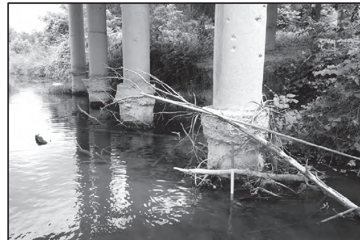
BENT NO. 7 LOOKING SE
