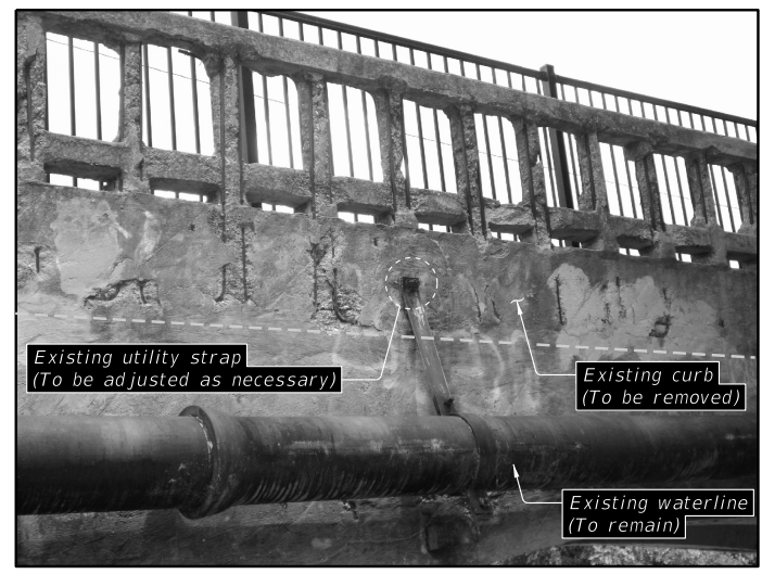
UTILITY SUPPORT STRAP DETAIL
