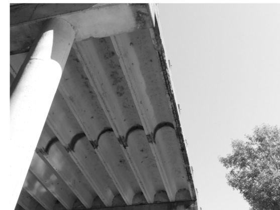
SP-3 (at Span 3)
