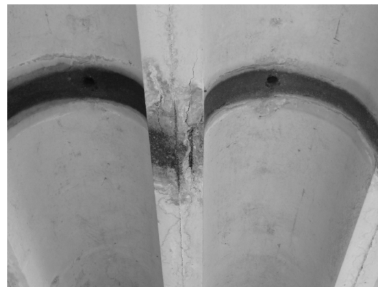
SP-3 (at Span 1)
