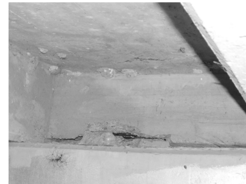
SP-1 (at Abutment 1)
