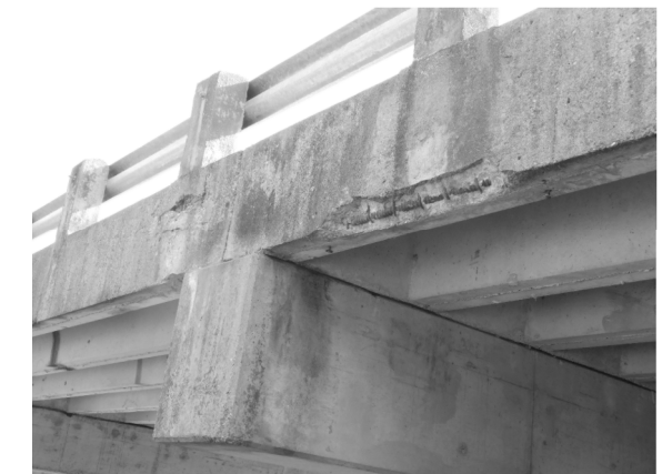
SP-3 (at Span 5)
