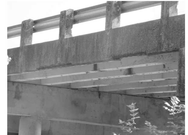
SP-3 (at Span 3)
