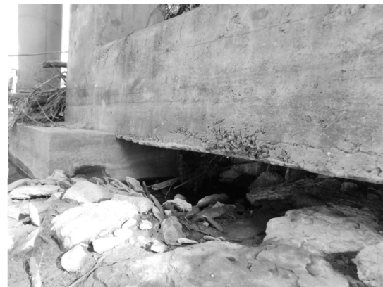
SB-3 (at Bent 4)
