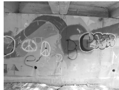
SB-1 (at Abutment 6)
