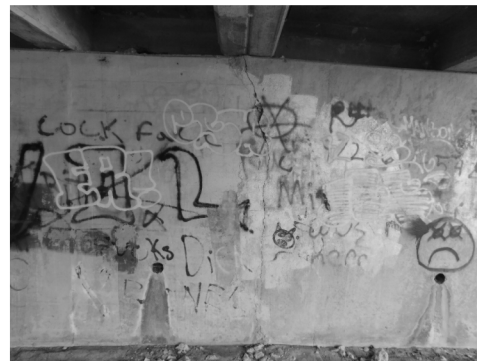
SB-1 (at Abutment 1)
