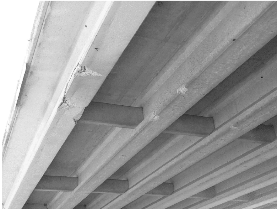
BEAM #1 DAMAGE Showing concrete beam repair and strand splicing locations. Remove enough concrete to provide adequate clearance for splices.
