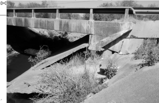
EROSION AND UNDERMINING OF RIPRAP AT SW CORNER LOOKING NORTHEAST
