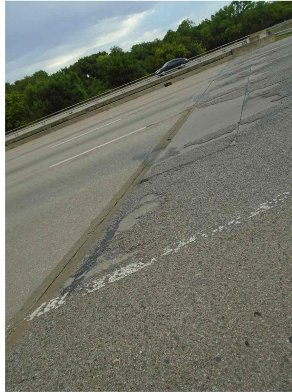
REPAIR D1207 EAST APPROACH SLAB LOOKING NORTH
