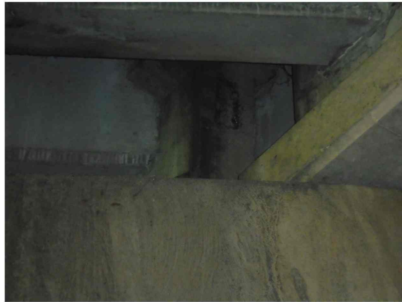
REPAIR SP1201 TYPICAL BEAM END LOOKING EAST
