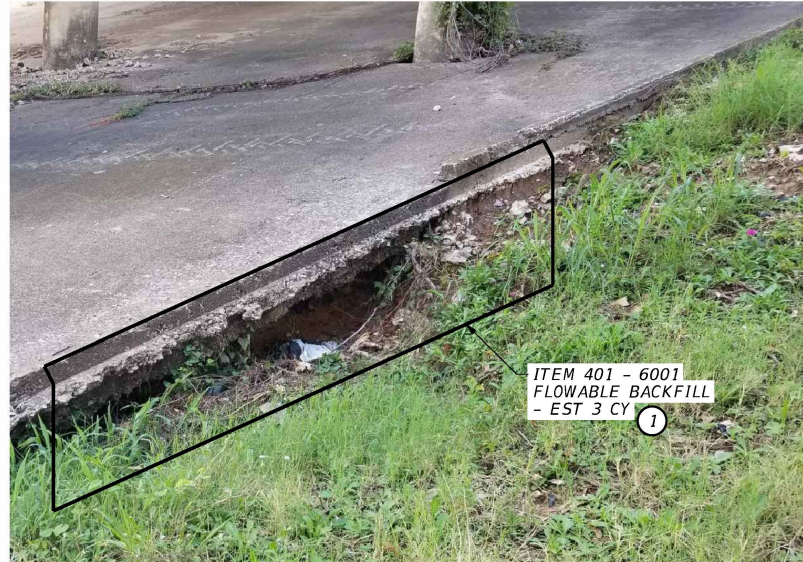
REPAIR M1901 UNDERMINING OF SW RIPRAP
