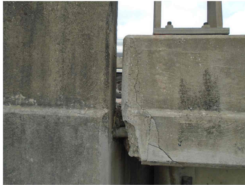
REPAIR D1302 ABUT 1 - DECK SPAN 1 INTERFACE LOOKING NORTH
