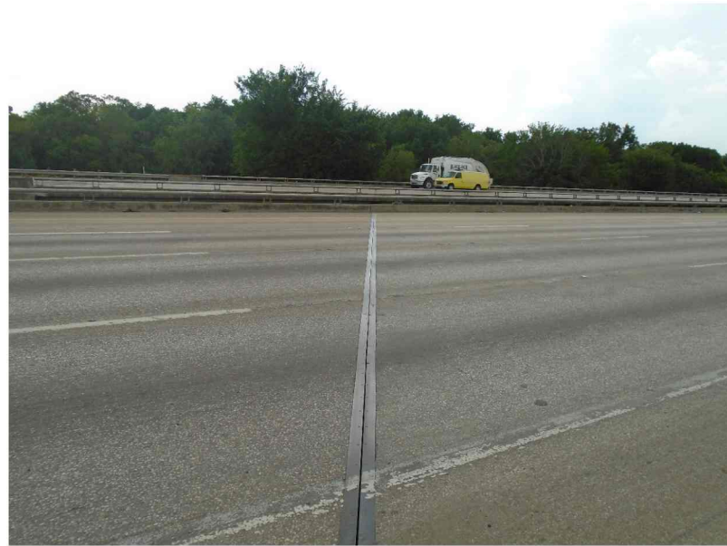
REPAIR D1301 BENT 7 EXPANSTON JOINT LOOKING SOUTH
