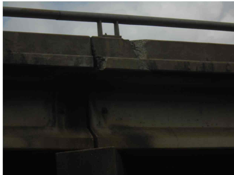
REPAIR D1304 DECK INTERFACE AT BENT 3 LOOKING NORTH
