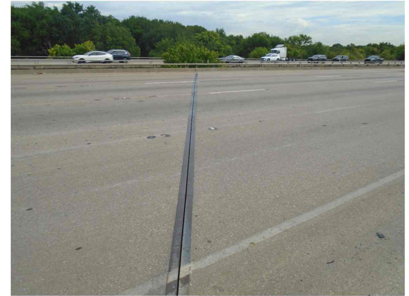
REPAIR D1201 BENT 4 EXPANSION JOINT LOOKING NORTH
