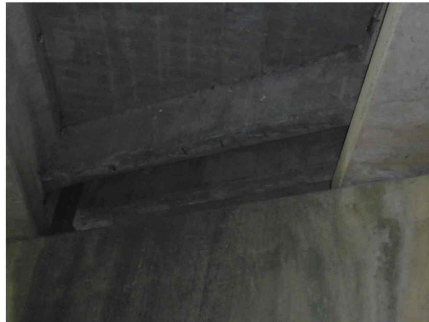
SB1305 BENT 3 BAY 5 DIAPHRAGM LOOKING WEST
