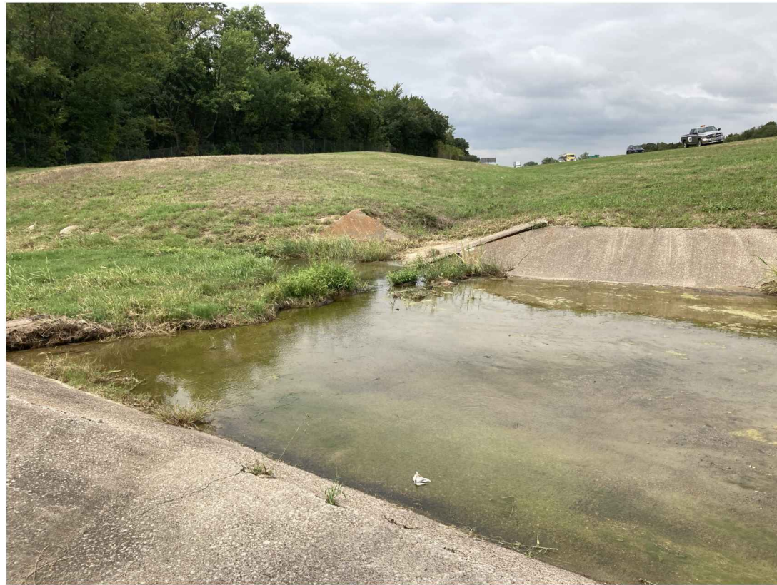
REPAIR M1401/M1402 SOUTH END RIPRAP REMOVAL AND REPLACEMENT
