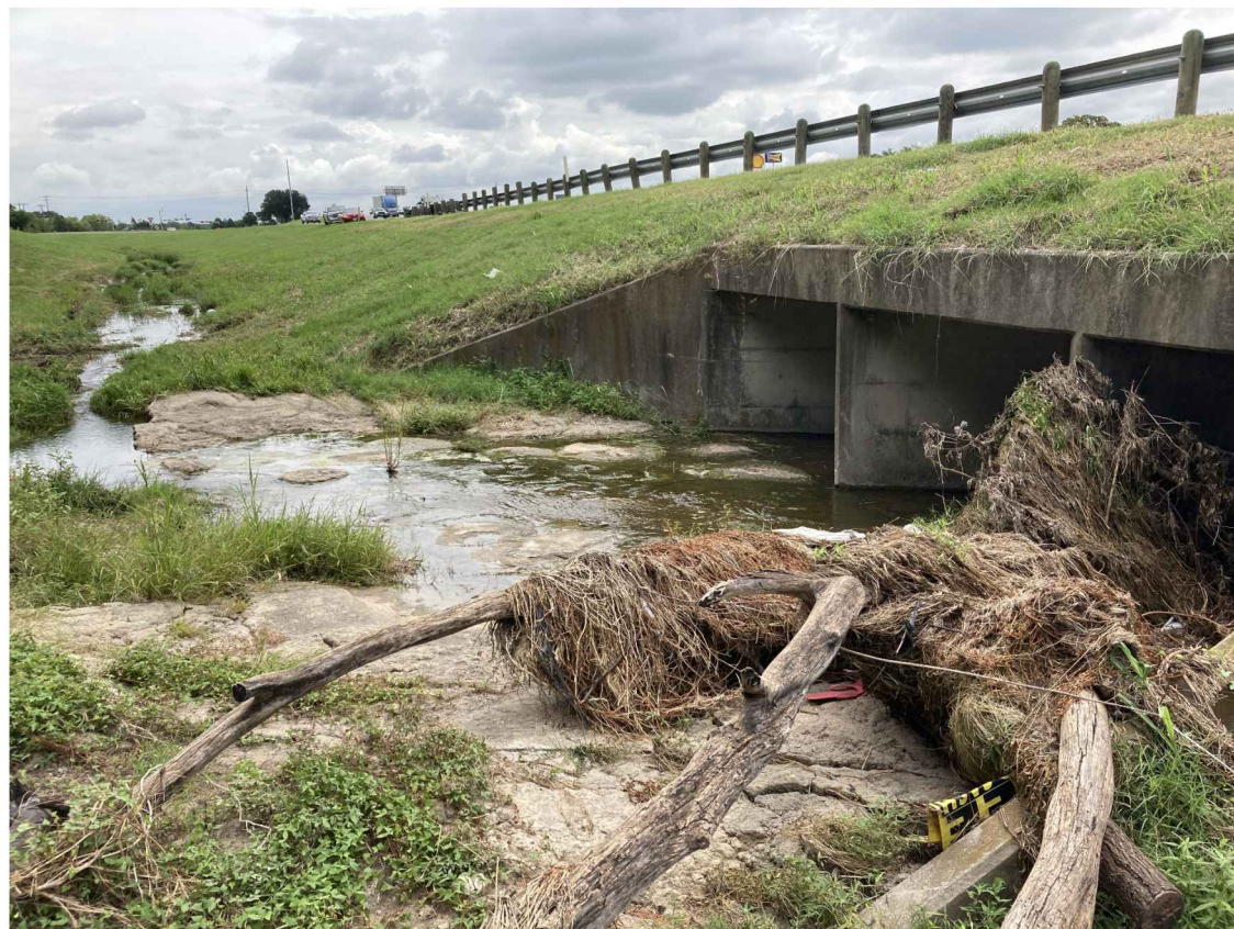
REPAIR M1404/M1405 NORTH END RIPRAP REMOVAL AND REPLACEMENT
