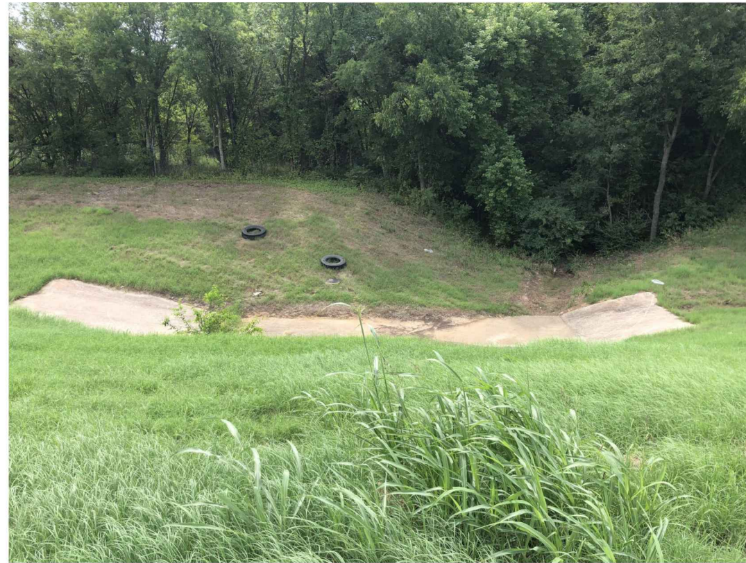
REPAIR M0702 SOUTH END APRON SRR
