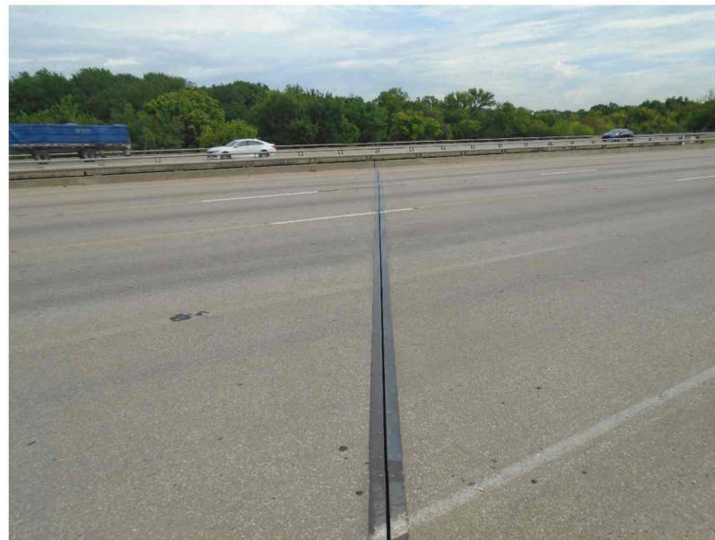
REPAIR D1201 BENT 6 EXPANSION JOINT LOOKING NORTH
