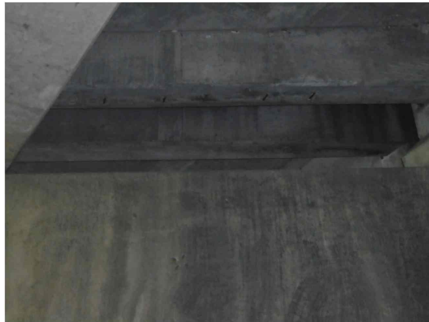
SB1304 BENT 3 BAY 4 DIAPHRAGM LOOKING WEST
