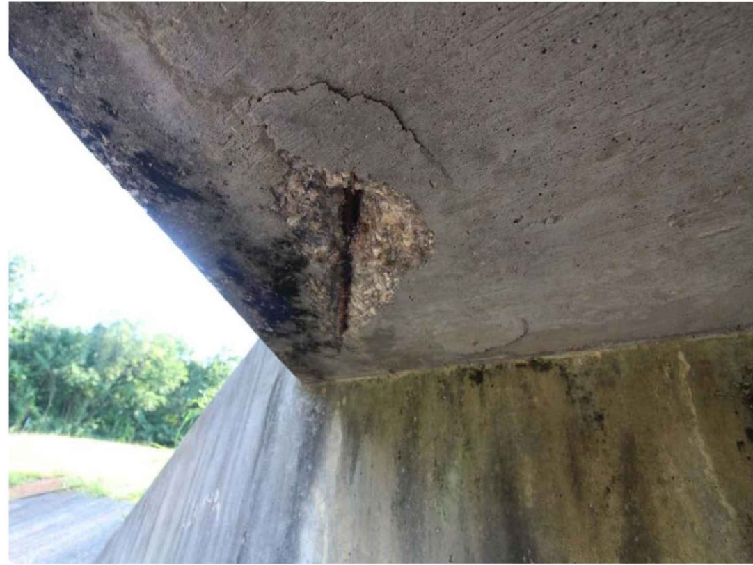
REPAIR SB1401 SOUTH END TOP SLAB SPALL
