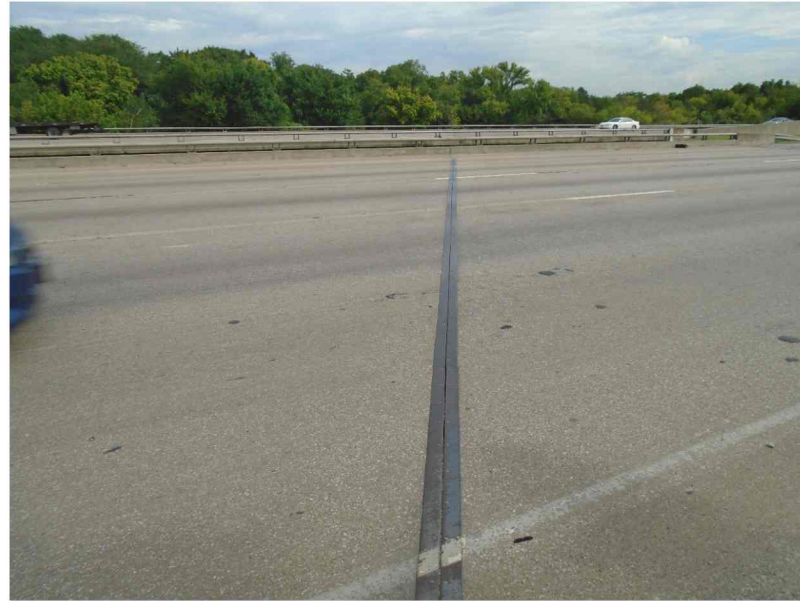
REPAIR D1201 BENT 7 EXPANSION JOINT LOOKING NORTH
