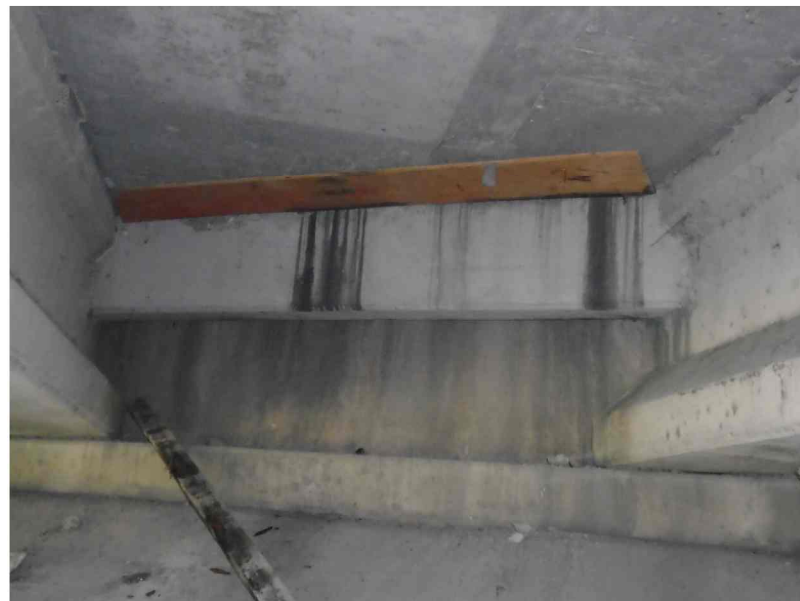
REPAIR SB1203 ABUTMENT 8 BACKWALL LOOKING EAST (SUBSIDIARY TO ABUTMENT BACKWALL REPAIR)
