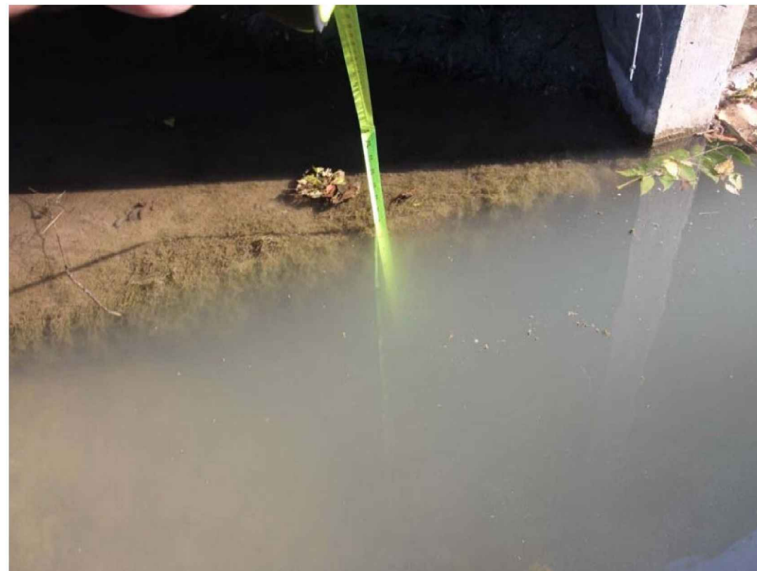
REPAIR M0601/M0602 TOE SCOUR AT SOUTH END
