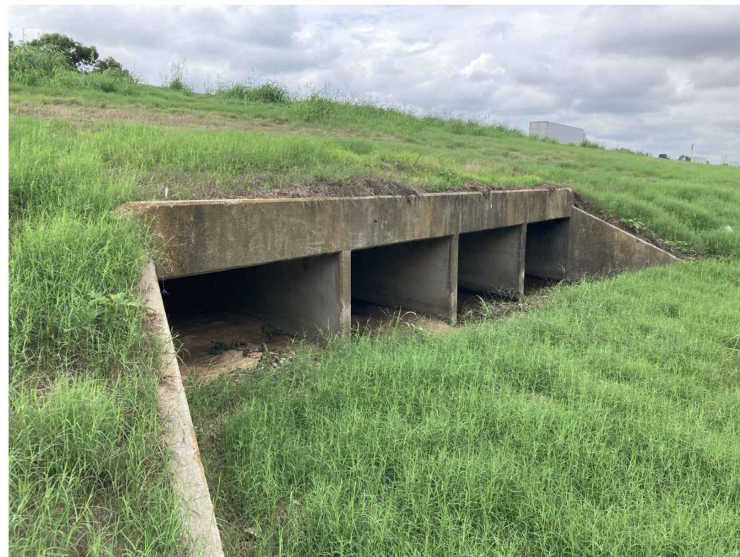
REPAIR M0703 NORTH END DEBRIS AND SILT
