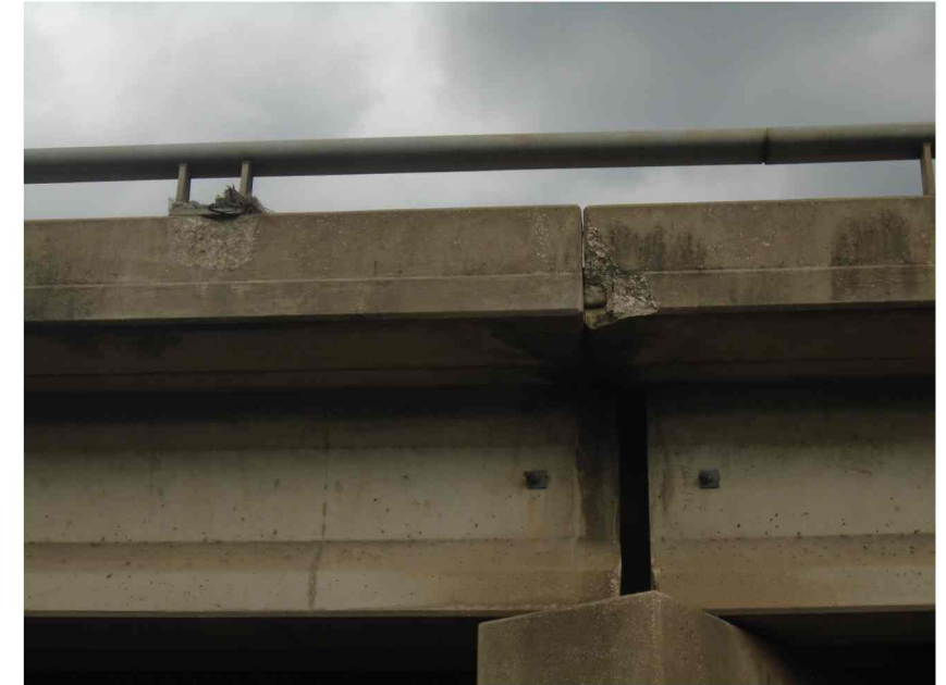
REPAIR R1301 BRIDGE RAIL LOOKING SOUTH
