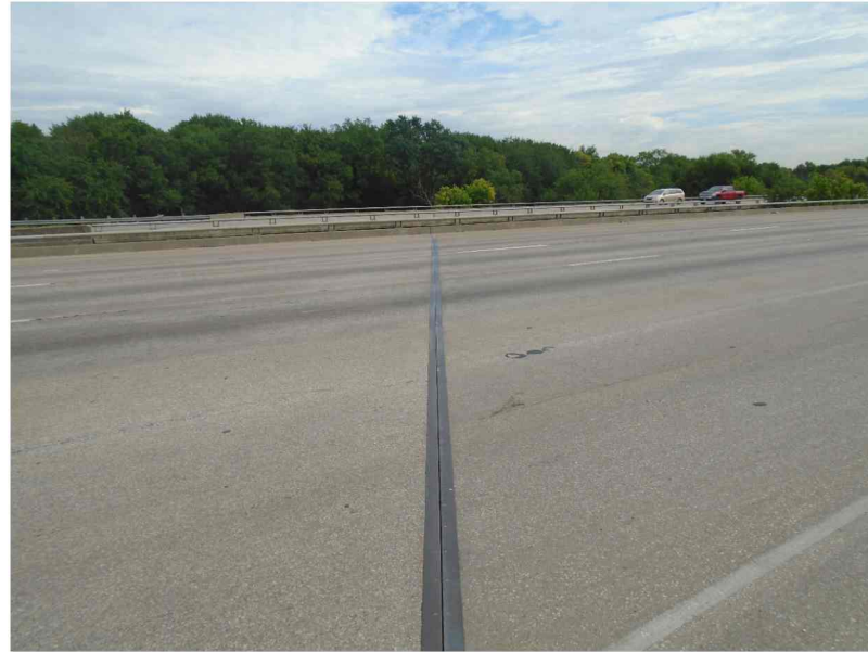
REPAIR D1201 BENT 2 EXPANSION JOINT LOOKING NORTH
