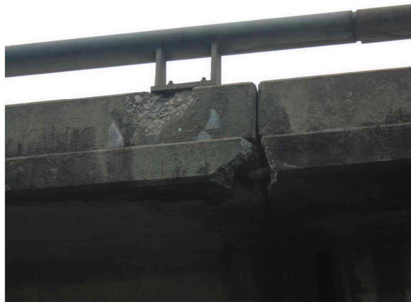
REPAIR D1205 BENT 3 SOUTH SIDE LOOKING NORTH
