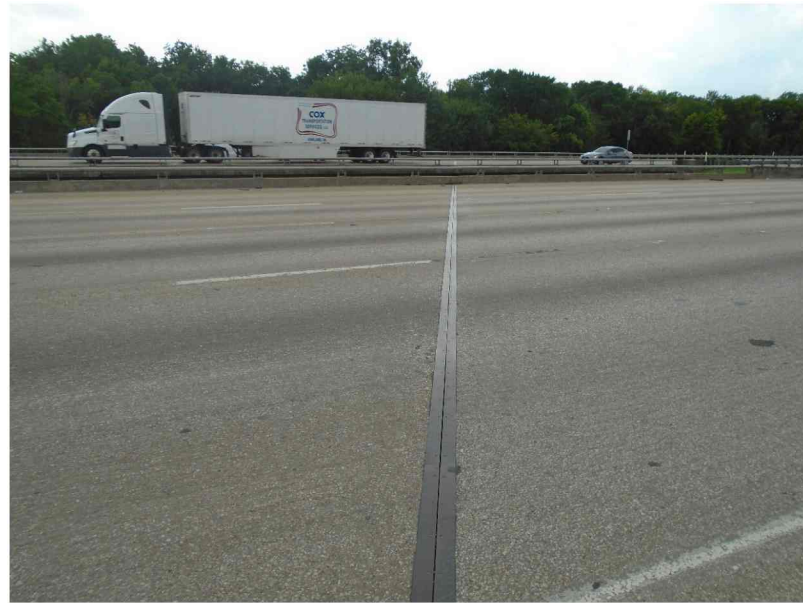
REPAIR D1301 BENT 2 EXPANSTION JOINT LOOKING SOUTH
