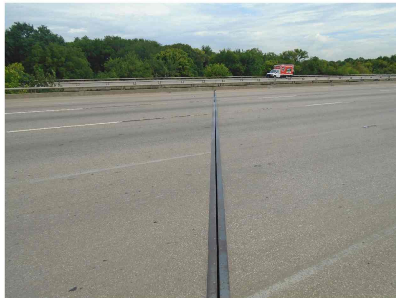
REPAIR D1201 BENT 5 EXPANSION JOINT LOOKING NORTH
