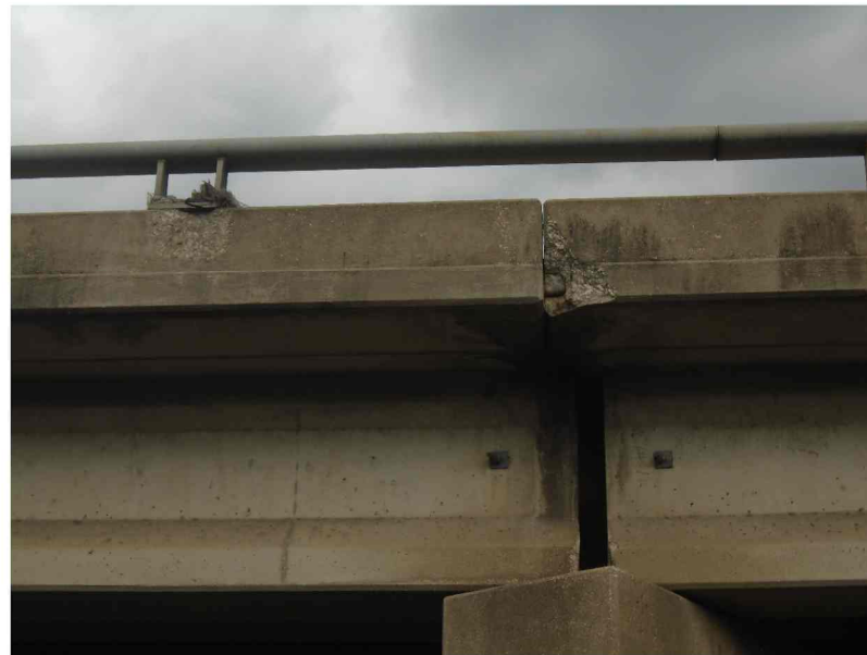
REPAIR D1305 DECK INTERFACE AT BENT 7 LOOKING NORTH
