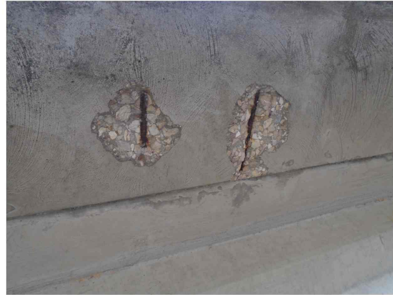
REPAIR D1202 SPAN 1 DECK SOFFIT NORTH SIDE FROM BELOW
