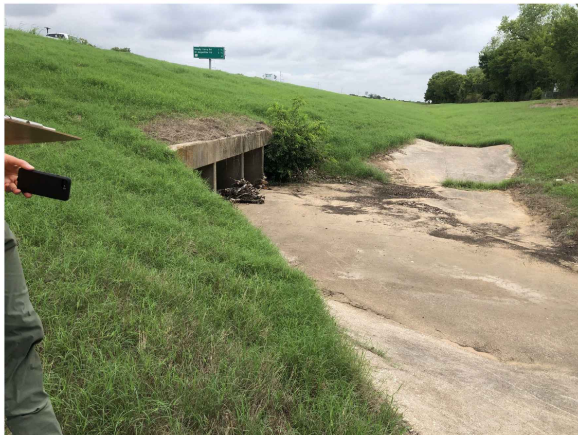
REPAIR M0703 SOUTH END APRON DEBRIS
