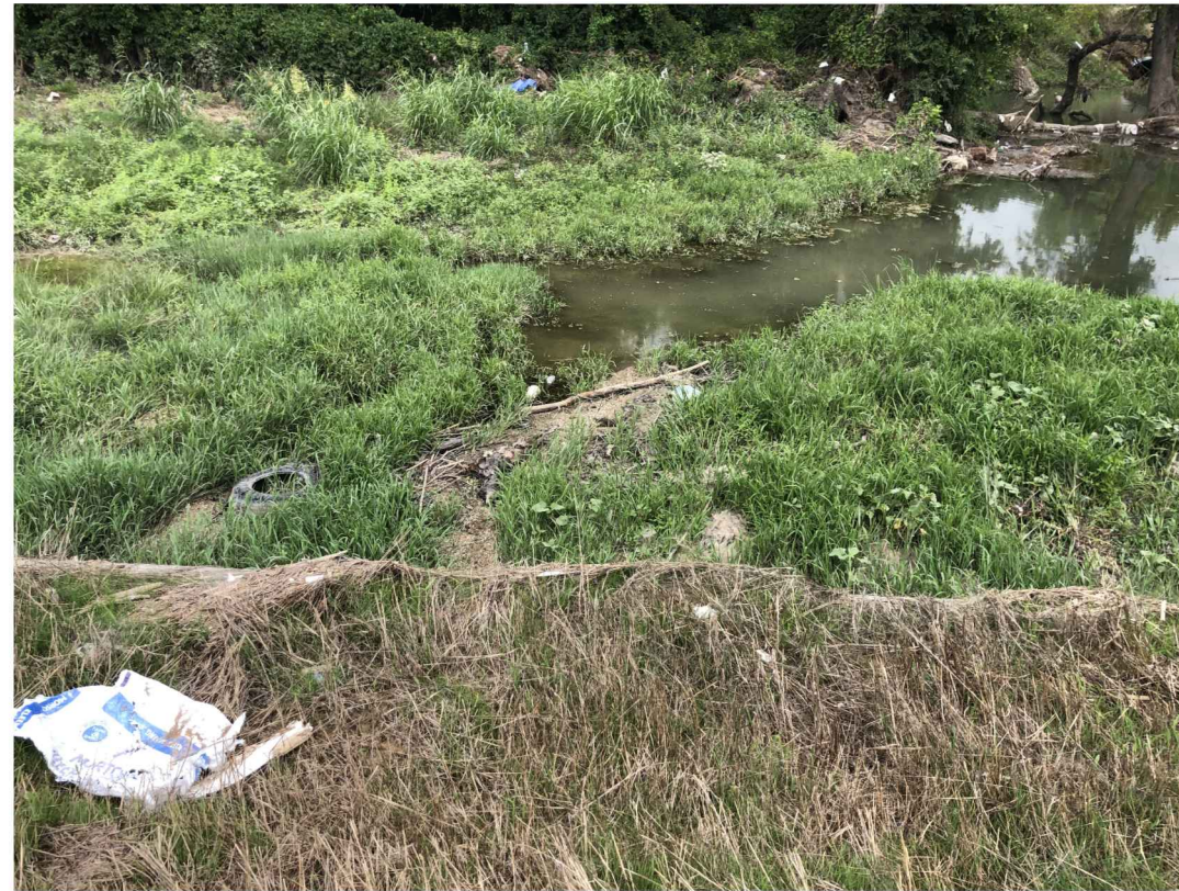
REPAIR M0603 NORTH END OF CULVERT
