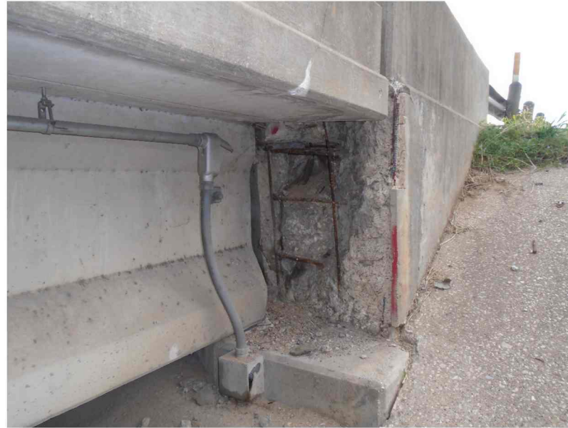
REPAIR SB1202 SOUTH END OF ABUT 8 BACKWALL LOOKING EAST
