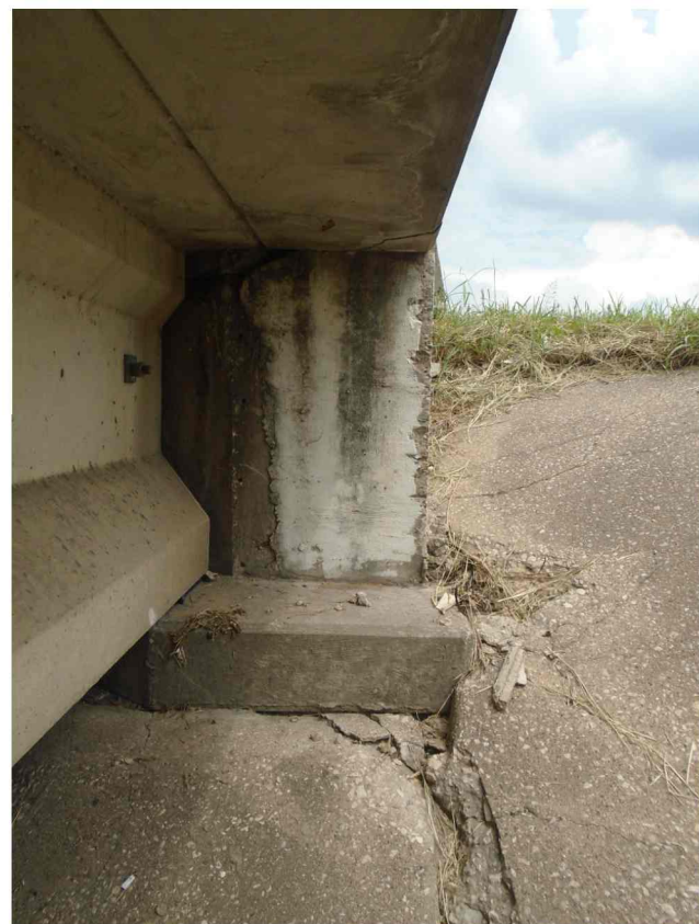
M1301, M1302, & M1303 ABUT 8 RIPRAP SOUTH END LOOKING EAST
