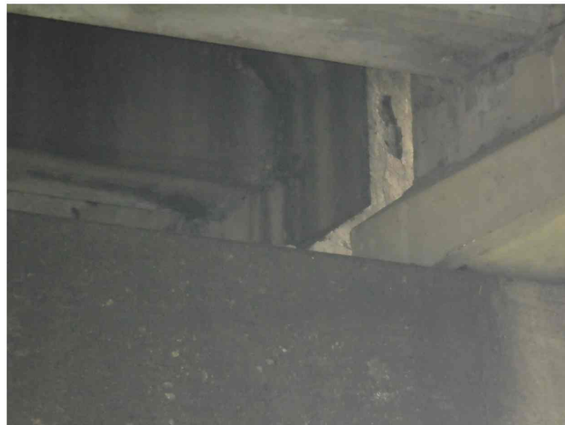
REPAIR SP1301 GIRDER END LOOKING EAST
