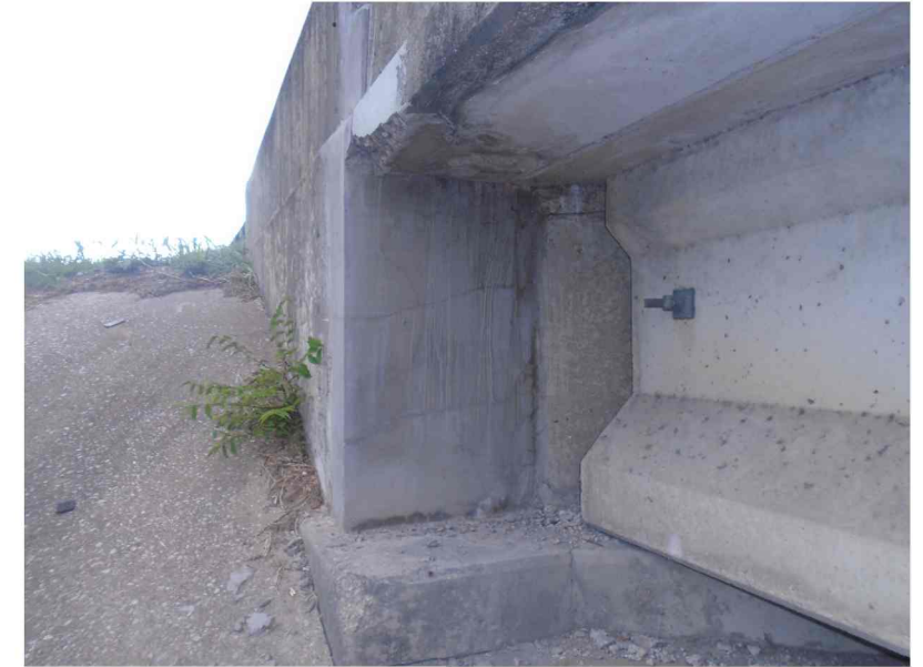
REPAIR SB1203 NORTH END OF ABUT 8 BACKWALL LOOKING EAST
