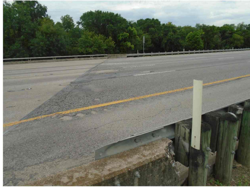
REPAIR D1207 WEST APPROACH SLAB LOOKING SOUTH
