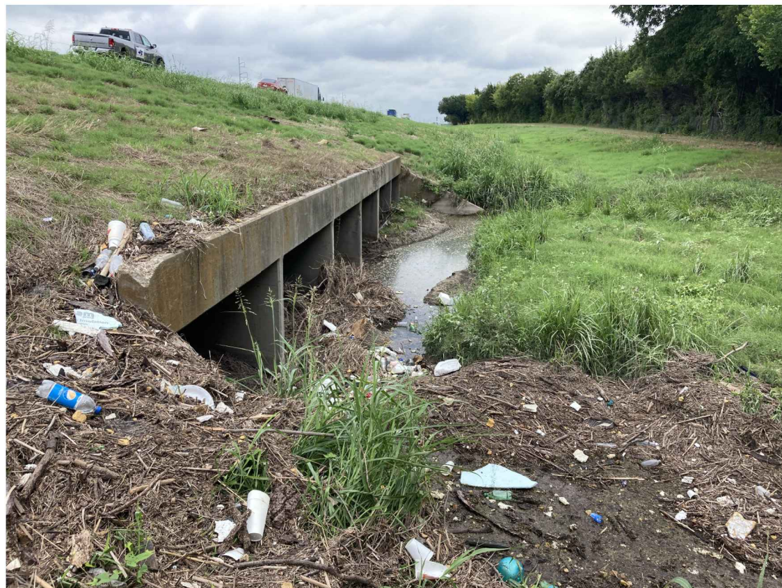
REPAIR M0603 SOUTH END OF CULVERT
