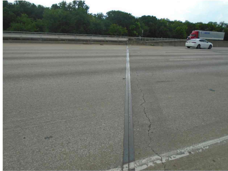
REPAIR D1306 ABUT 1 APPROACH SLAB LOOKING SOUTH
