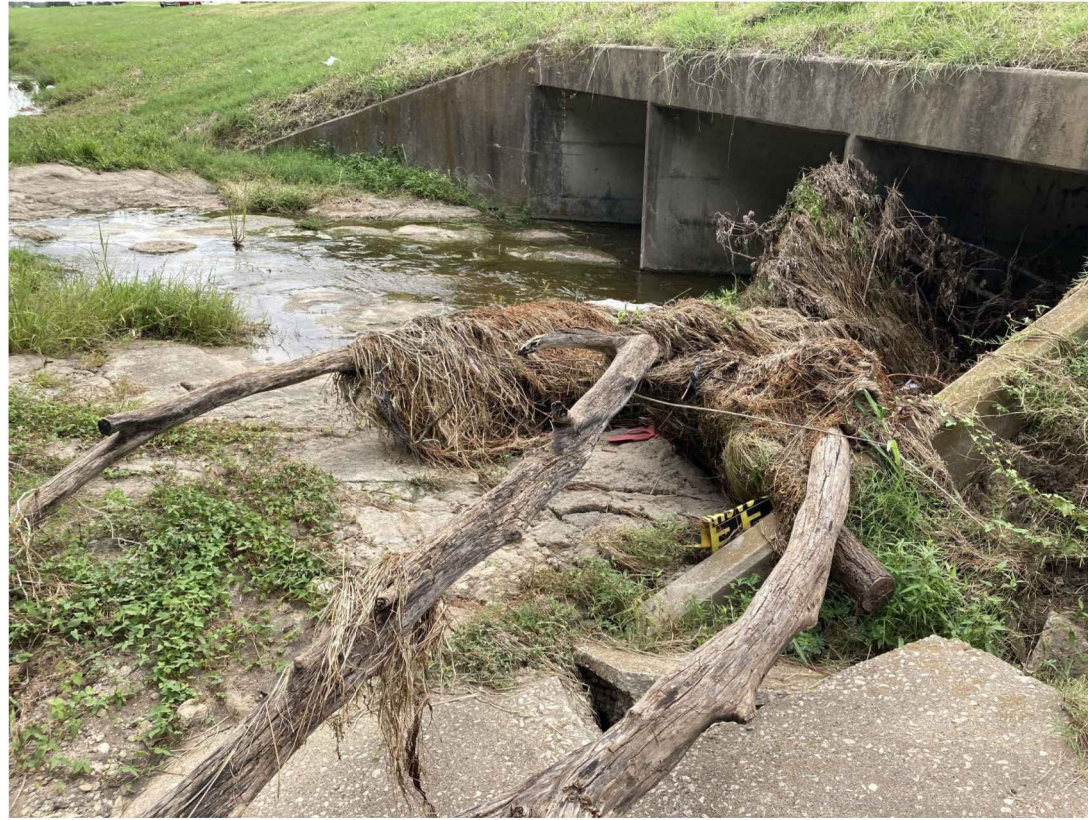
REPAIR M1407 NORTH END DEBRIS REMOVAL
