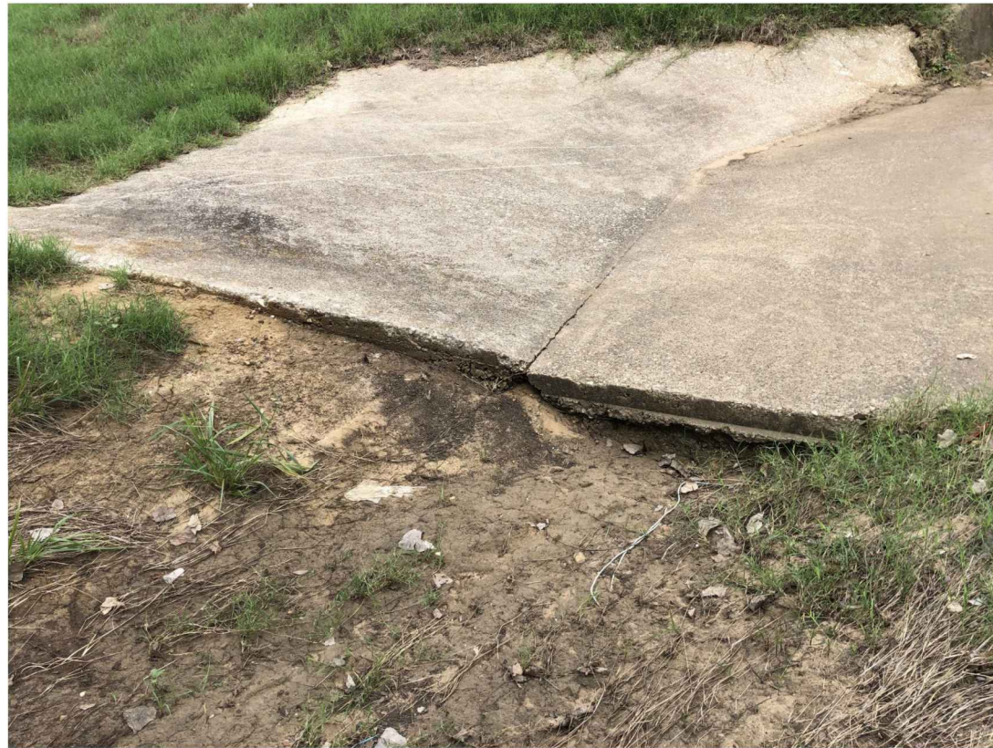
REPAIR M0701/M0702 SOUTH END APRON SLAB SCOUR
