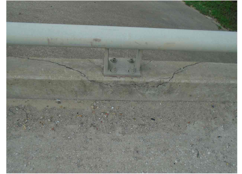
REPAIR R1201 TYPICAL STRUCTURAL RAIL LOOKING SOUTH
