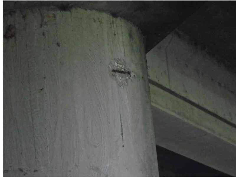
REPAIR SB1201 BENT 7 COLUMN 2 LOOKING WEST
