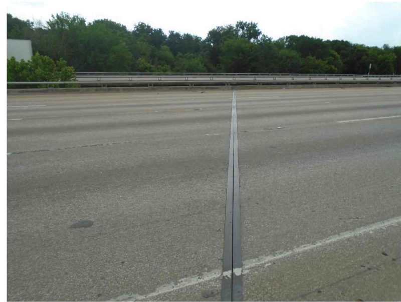
REPAIR D1301 BENT 3 EXPANSTION JOINT LOOKING SOUTH
