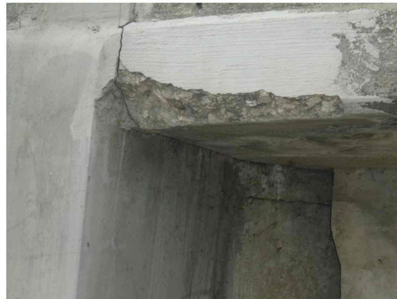
REPAIR D1206 ABUTMENT 8-DECK INTERFACE NORTH SIDE LOOKING SOUTH
